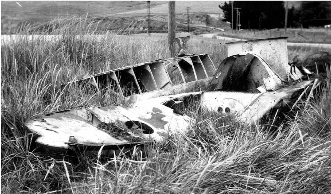
Figure 70. Remnants of the torpedo boat Defender at Purau Beach, ca. 1941. The stern and midships section (with intact conning tower) are in the foreground. The bow section behind it is lying on its side. Image courtesy of the Alexander Turnbull Library, National Library of New Zealand (Accession No. F-66786-1/4).
