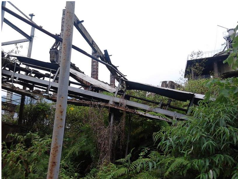
**Figure 1.2** Steel framed building in ChuanXinDian Chemical Park in Shifang County, suffered heavy damage during the 2008 Sichuan earthquake in China. Source: [https://commons.wikimedia.org/wiki/File:Shifa\\_Chuanxindian\\_earthquake\\_park\\_05.jpg](https://commons.wikimedia.org/wiki/File:Shifa_Chuanxindian_earthquake_park_05.jpg), via Wikimedia Commons.
