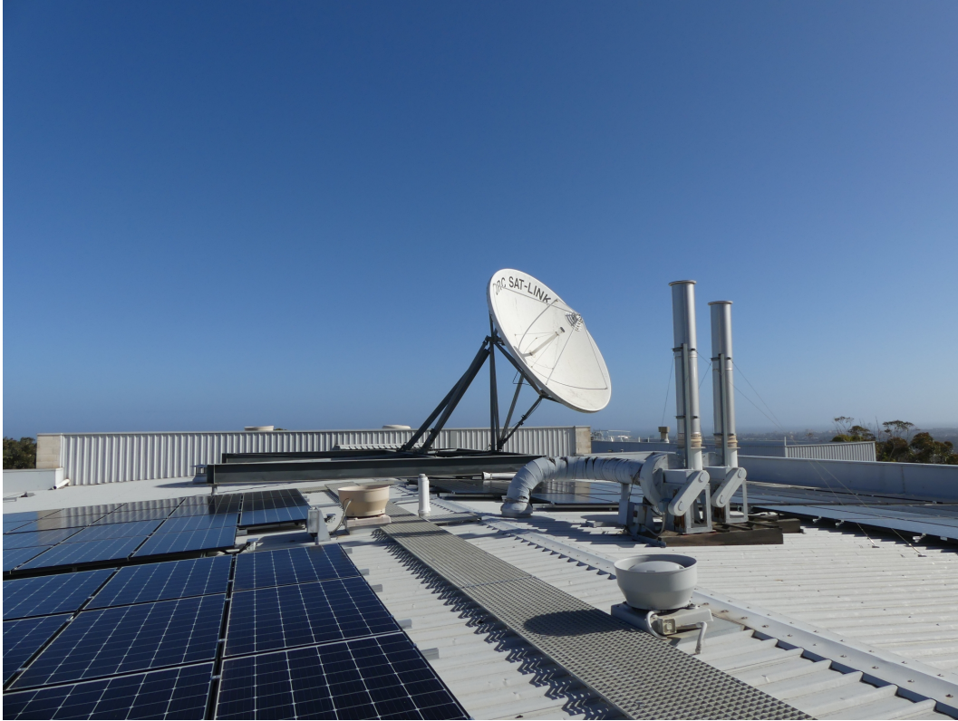
FIGURE 10.6: A 20 years old satellite 4.5m diameter dish already installed at Flinders University-Bedford campus has been employed to up-link data to the satellite, then broadcast data to other remote communities. Considerable work was required to recommission this dish to act as a ground-station
