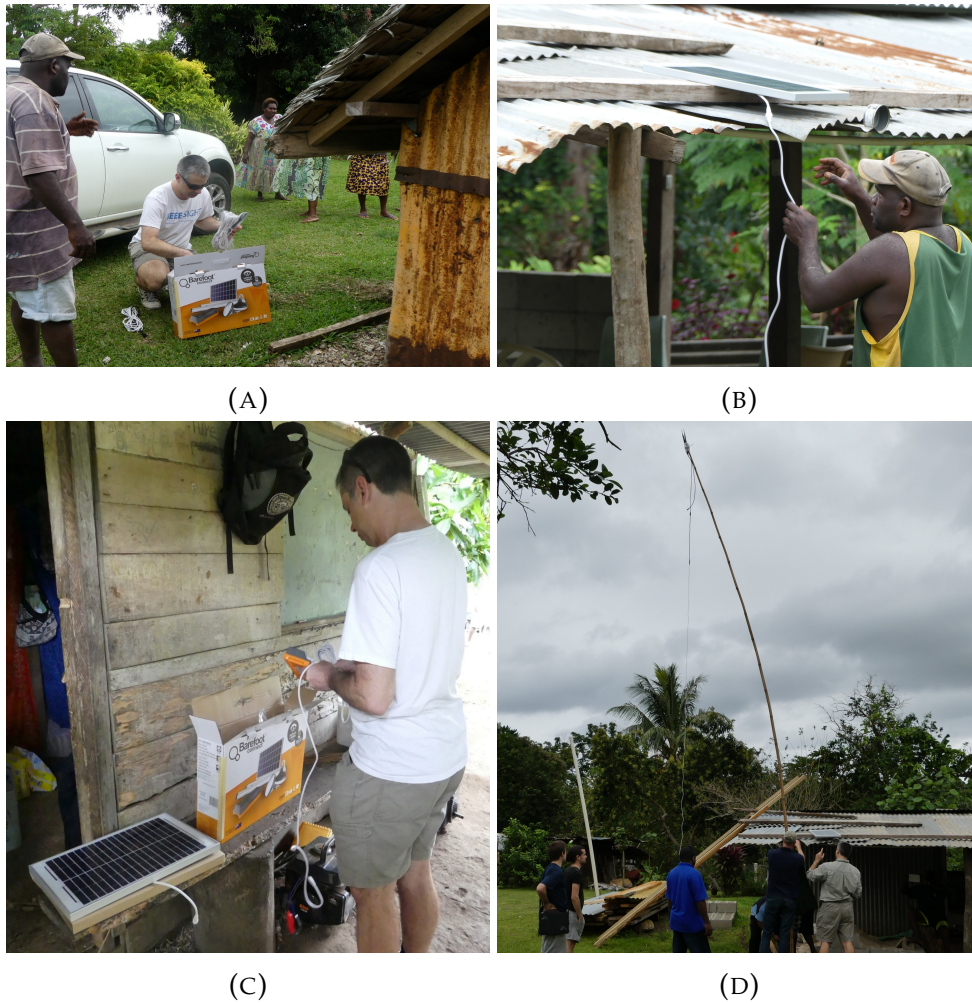
FIGURE 8.4: Installing solar panel to provide power for Serval Mesh Extenders in the village of Pang Pang in Vanuatu, as part of the pilot of the Serval Mesh in Vanuatu. This village lacks access to the national electricity grid, despite being located on the main island of Vanuatu. Such situations are common, because of the small populations in these villages, which are often separated by many kilometres from one another.
