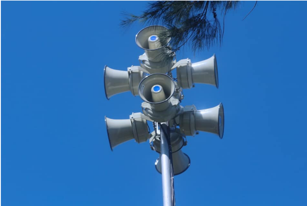
FIGURE 10.1: The upper section of a tsunami early warning siren tower in Dili, Timor Leste (Image in the public domain). These towers are typically 20 to 50 metres in height, are expensive to install, and expensive and complex to maintain in remote Pacific Island Nation contexts, especially where they are faced with regular cyclones and a highly corrosive tropical maritime environment.
