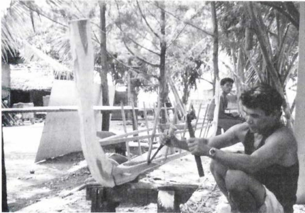
Figure 4-8. Frame-first construction of a Philippine banca (Aguilar 2006:73).
