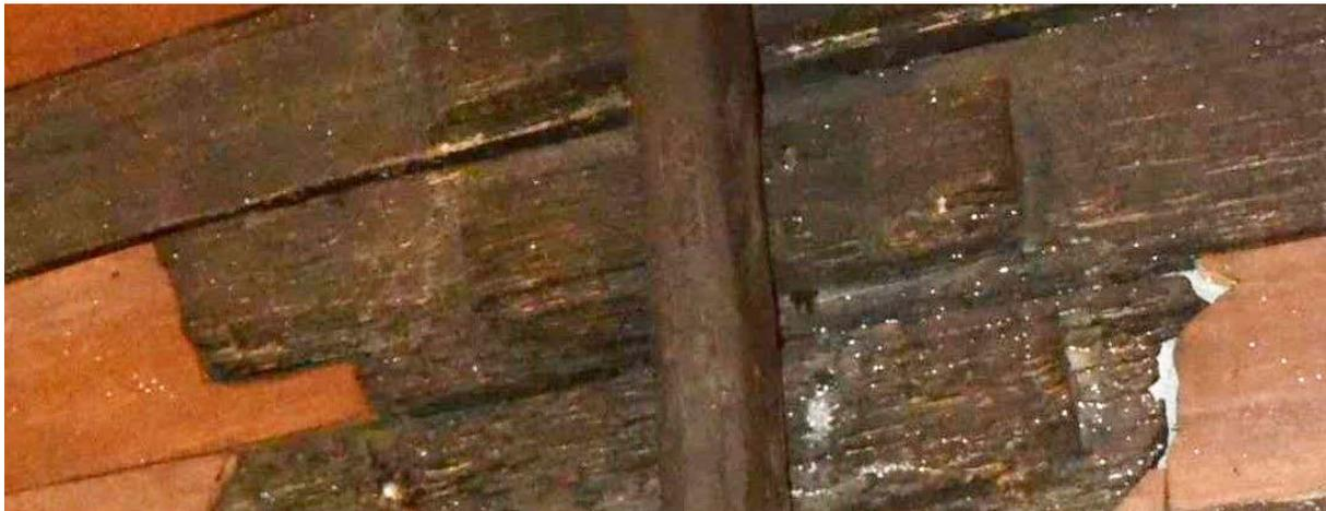
Figure 6-33. Second plank of Butuan Boat 2 STR-B4 near last lug. Photograph by author.
