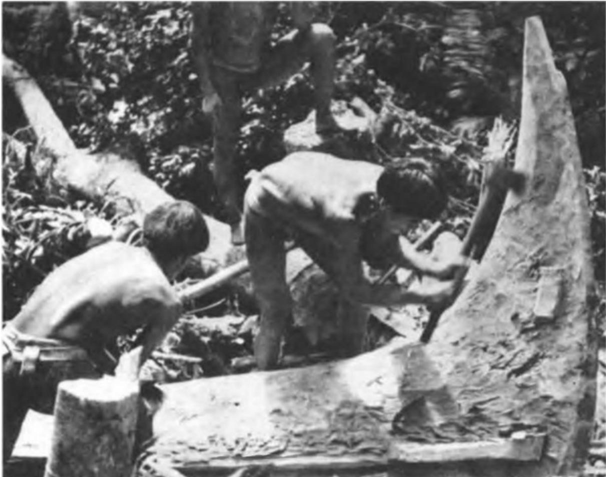
Figure 4-15. Yami boat showing buttress root sheer strake plank. (Kano and Segawa 1956:301).
