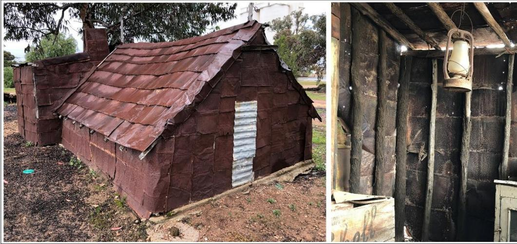
Figure 7.28 House at Poochera, Eyre Peninsula, built in the 1920s from flattened kerosene tins and poles cut from local pine trees. Photos: Susan Arthure.
