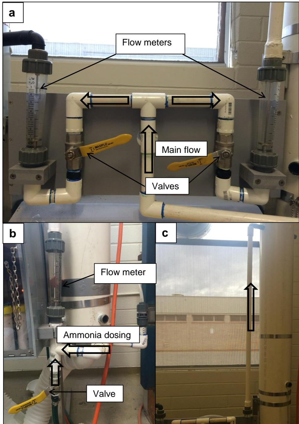
**Plate 2.6** PVC manifold: (a) the main flow and two branches; (b) the main flow and the ammonium dosing line; (c) influent line for one of the filters.
