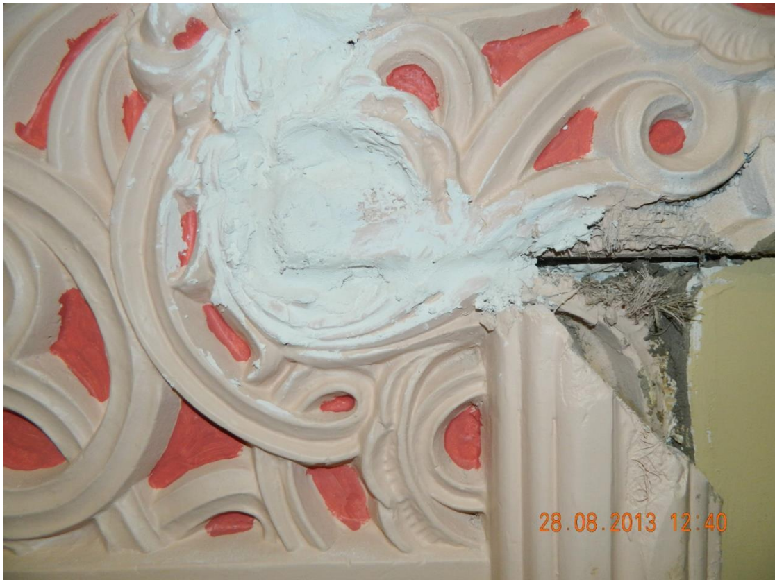
Figure 5.18. Damage to and attempted repairs on decorating side panelling of the Vogue. The building has sustained damage from natural deterioration through the years. Taken by author.
