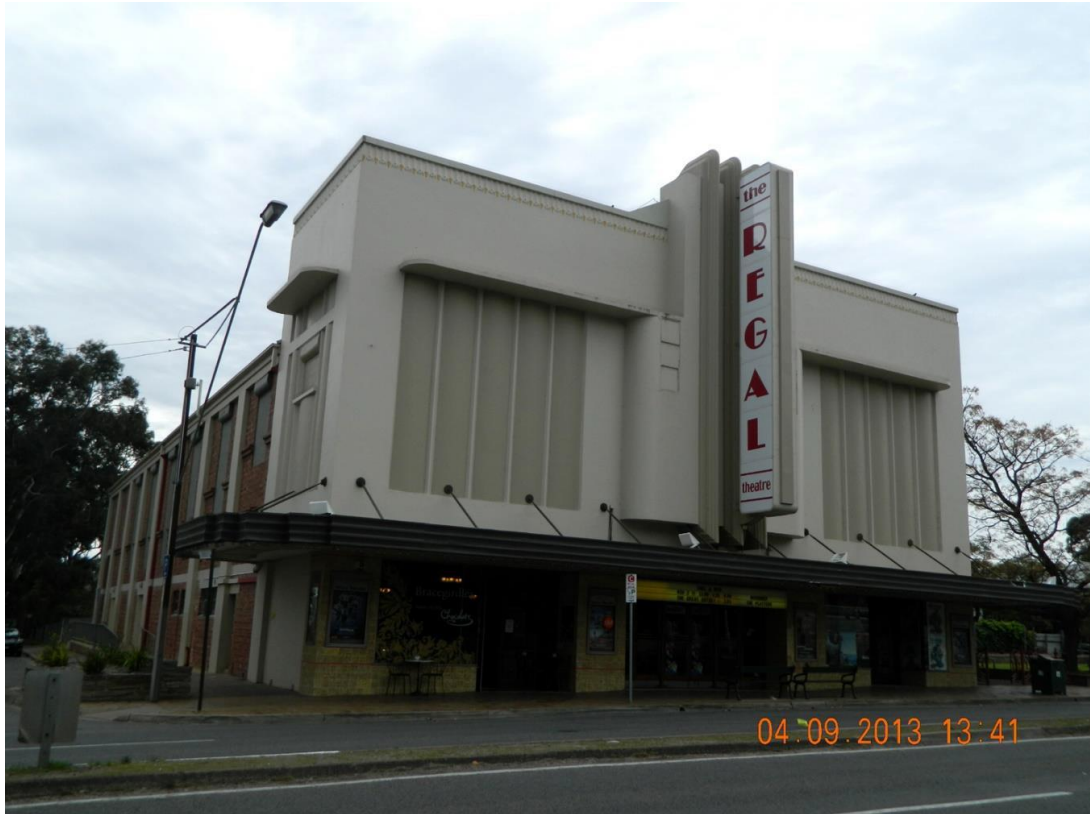
Figure 5.16. Facade of the Princess Theatre (now The Regal), Marryatville. It was renovated in the 1940s into its current design. Taken by author.
