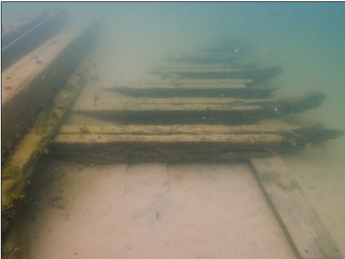
Figure 4.8: Image of portside frame and keelson structure on Vessel A (La Barre 2015).
