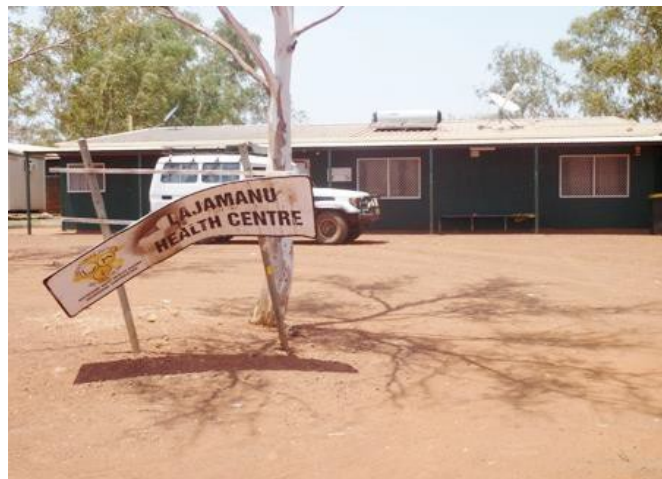
Old Health Centre (a new centre has since been built).
