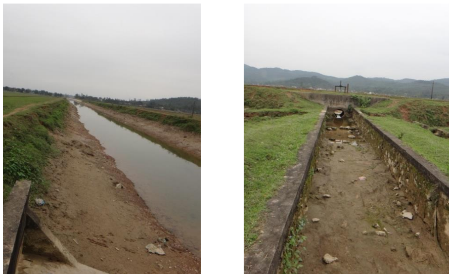
Figure 7-2: The main canal and the headwork of the N6 secondary system
