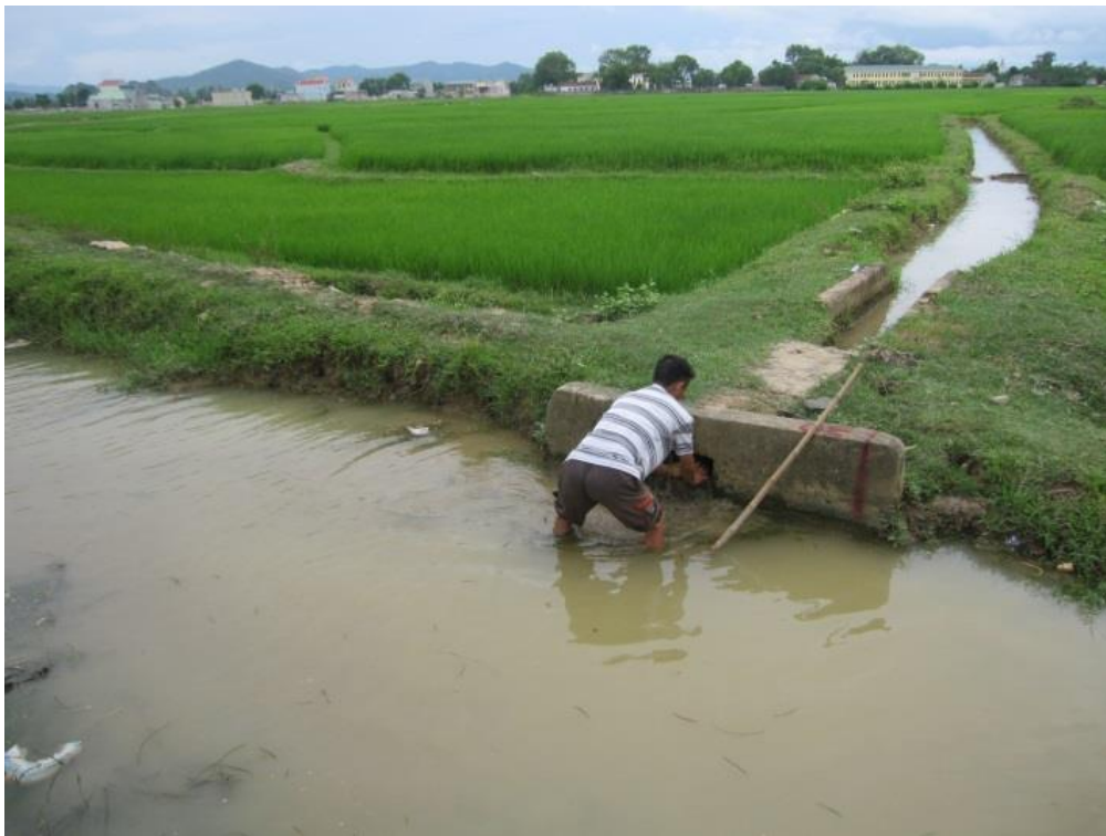
Figure 7-10: Irrigator closing the offtake by filling canal with soil, 2013
