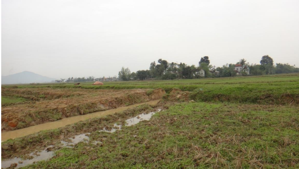
Figure 7-11: Earthen secondary canals
