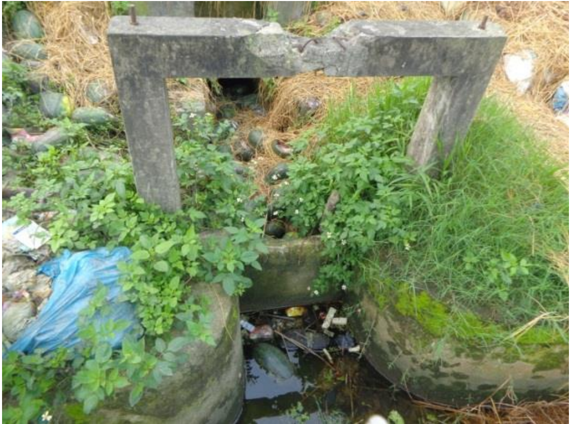
Figure 6-13: Watermelon and straw blocking canals in Gia Xuyen system
