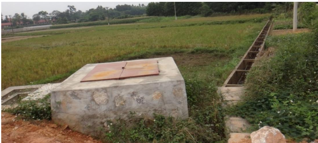
Figure 5-8: Concreted secondary canal systems with manual off-take in Ngoila
