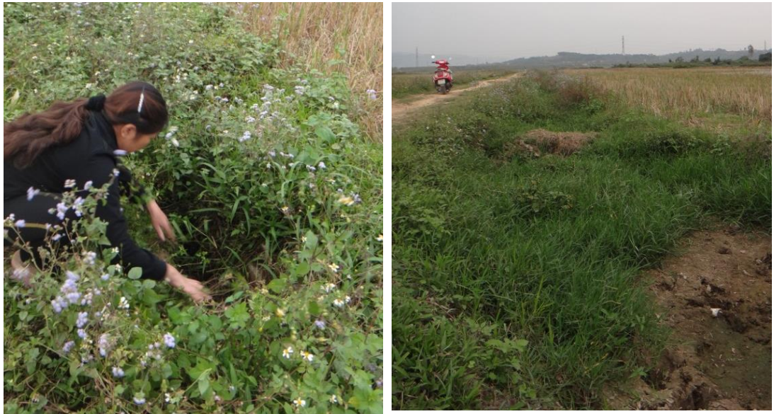
Figure 5-12: Former staff of WUA show the degradation of on-farm irrigation systems at Kim Phu commune
