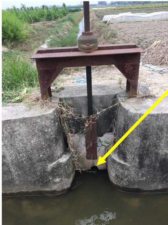
Figure 6-9: Modified offtake of one of the secondary canals
