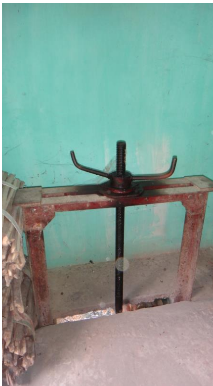
Figure 5-10: Protected water valve controls water
