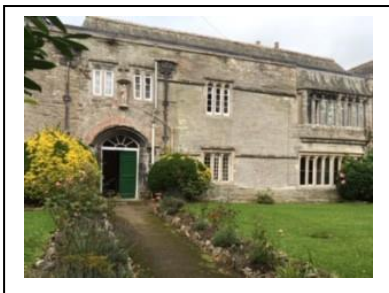
Part of the sixteenth century wing at Lanherne, which is now the front of the house. Photo taken by the author, Sept. 2016.
