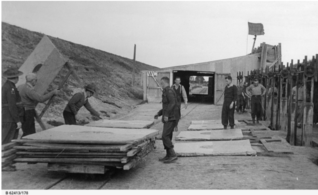
Figure 59. Target practice structures at Port Adelaide rifle range, 1942. (Source: State Library of South Australia B62413/178)
