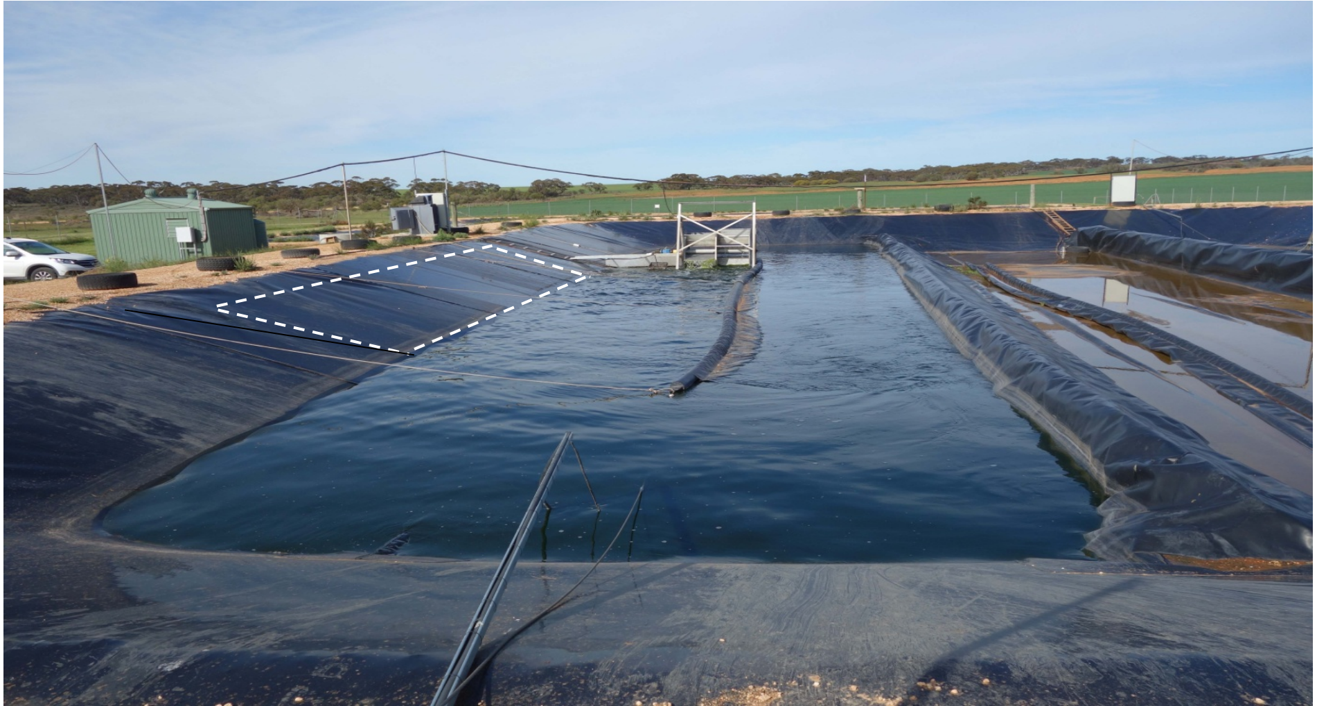
Plate 6.1: Example of the available freeboard for exposure on the HRAP at KoM. Surface area of the freeboard between the causeway and the start of the pond bend in the foreground was 52 m 2 . Estimate was generated with a 0.32 m depth pond.
