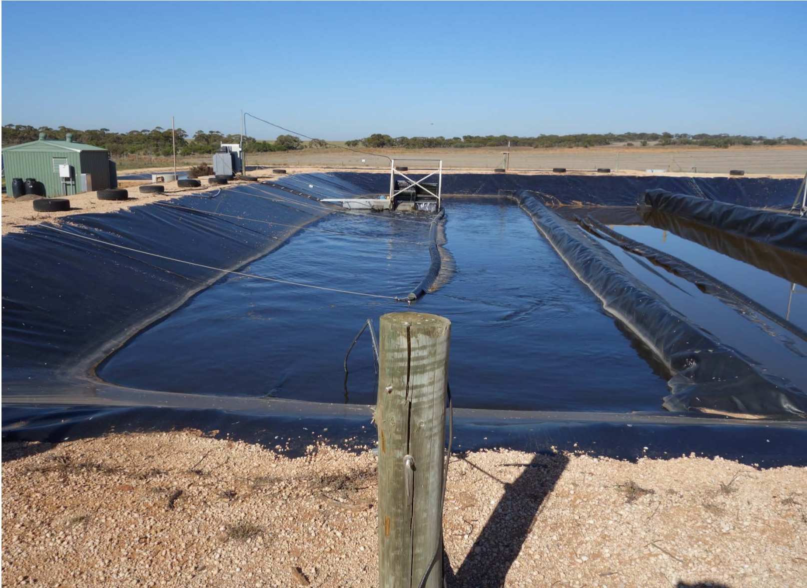
Plate 1.1: The inclined plane surrounding the high rate algal ponds (HRAPs) at Kingston on Murray (KoM), South Australia.
