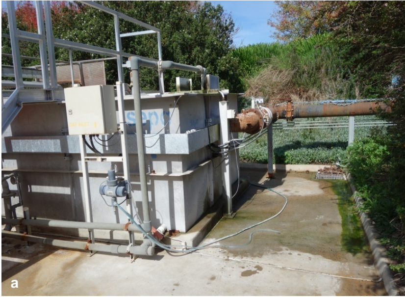
Plate 4.2: Pictures of the a) Dissolved air filtration (DAF) plant at Mt Barker wastewater treatment plant and b) inlet to DAF plant water sampling point
