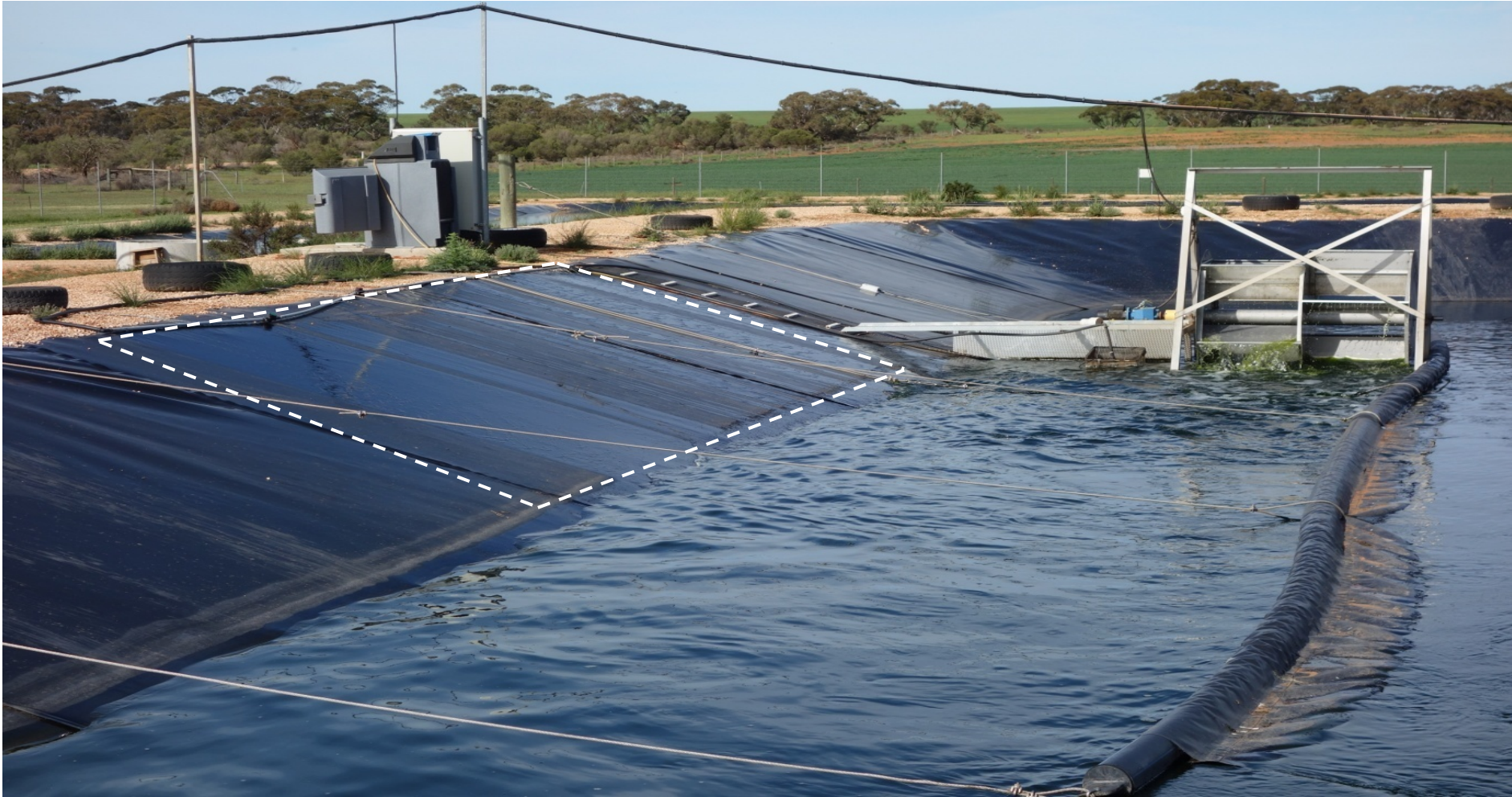
Plate 6.3: 36 m 2 IP (white rectangle) on the HRAP pond wall at Kingston on Murray (KoM), South Australia.
