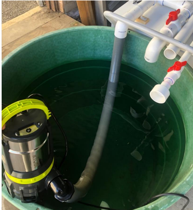
Figure 13. Connection of pump to flow cell
