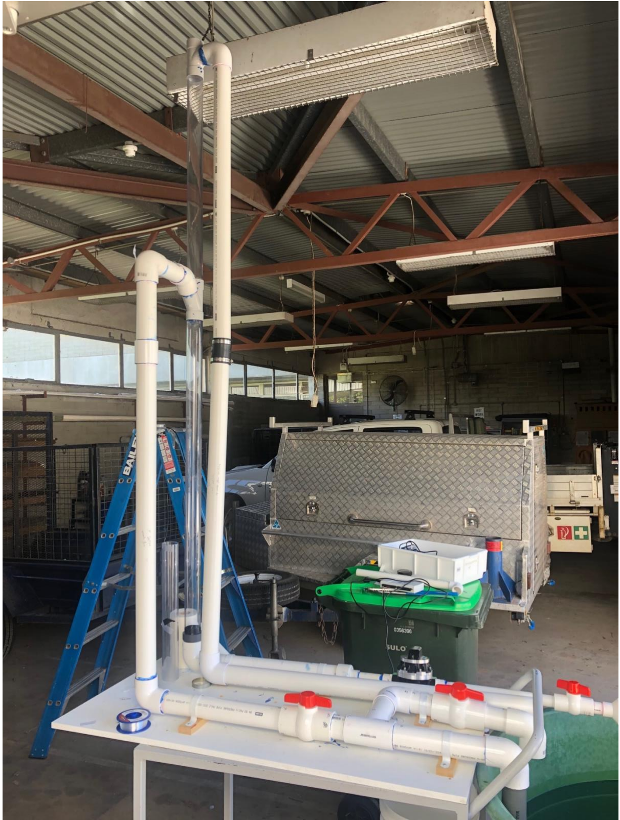
Figure 23. Side view of flow cell
