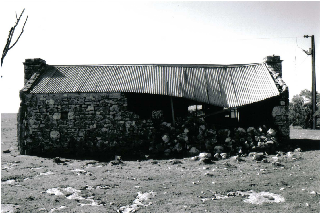
Figure 4.2.4. Recent (2005) photograph of the Men's Hut, showing the collapsed portion of wall on the western side.
