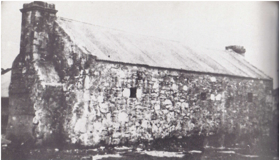
Figure 4.2.0. Western side of the 'Men's Hut' at Central Outstation. This photograph, taken in 1970, shows the appearance of this side of the building before the collapse of a large portion of the wall. Three rectangular apertures are clearly visible, evenly spaced along the wall. From Baillie, 1978: 134.
