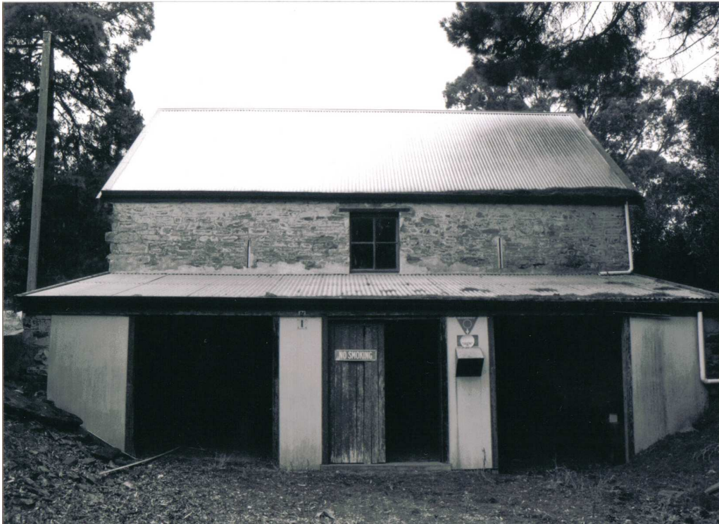
Figure 4.3.3. The western side of the coach-house. The apertures are visible on either side of the window, nearly half way between the window and the sides of the building, as narrow vertical slots.
