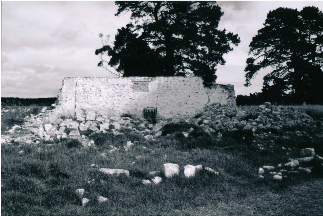
Figure 4.1.7. View of the western outbuilding at Mount Benson. The blocked up window can be seen in the upper centre of the wall, as can the rubble pile, evidently from the chimney, at right. The two large trees in the background are part of the avenue of trees believed to have marked the line of the old road. Facing south-east.
