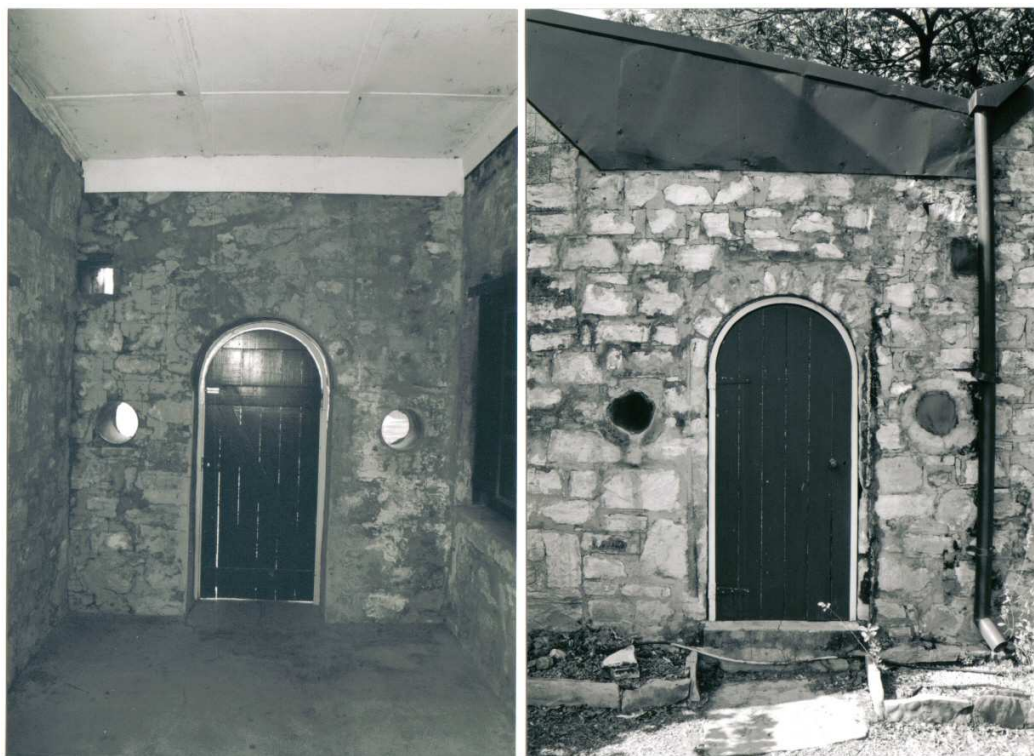
Figure 4.4.4. Interior (left) and exterior (right) of the northern door of the dwelling, showing the apertures built into the stonework.
