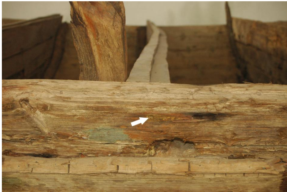
Figure 5-26 Square nail hole identified in the inner hull plank. Photo by author
