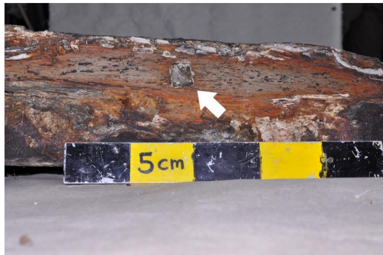
Figure 8-8 Cross-section of the nail remaining in the exposed seam. Photo by author
