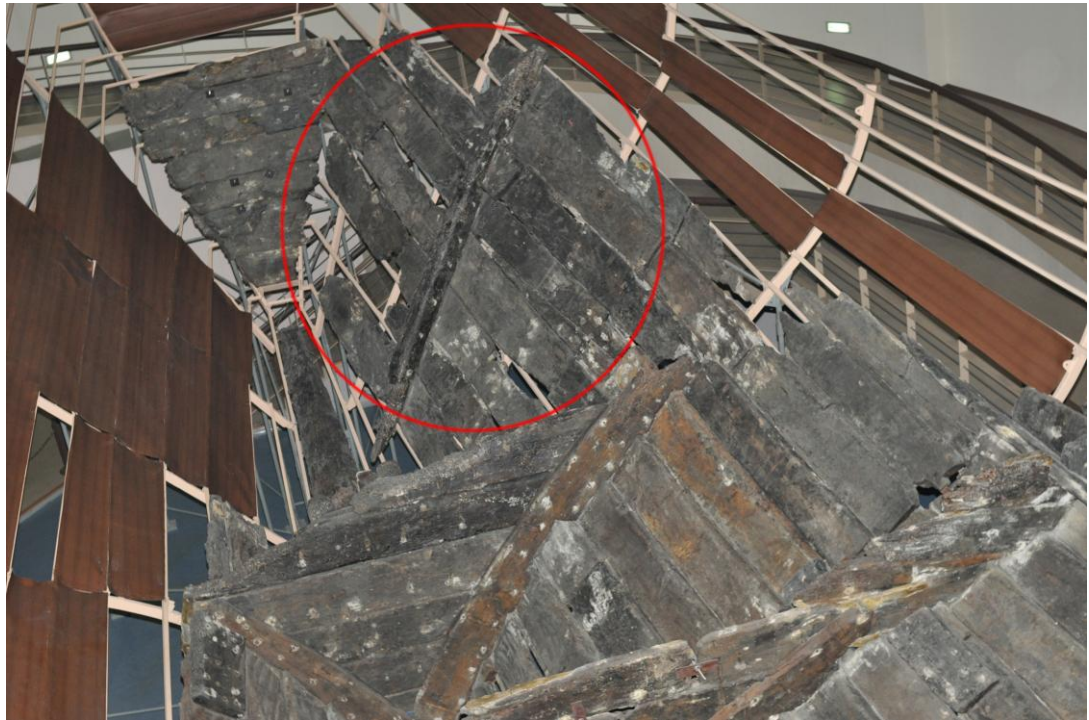
Figure 6-11 Baulk on the inside at the starboard in the bow. Photo by author
