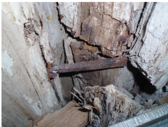
Figure 5-7 Modern iron nail seen at the bottom of the hull. Courtesy of Museum of Overseas Communication History
