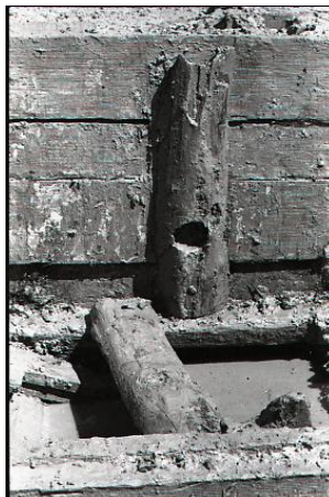
Figure 5-19 Bulkhead stiffener partially remains in the bottom of the hull. Courtesy of Museum of Overseas Communication History
