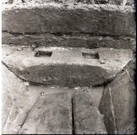
Figure 5-29 Old photograph of the forward mast step after excavated. Courtesy of Museum of Overseas Communication History
