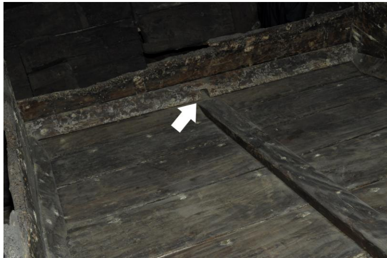
Figure 6-31 Photograph showing a drainage hole in the tank. Photo by author
