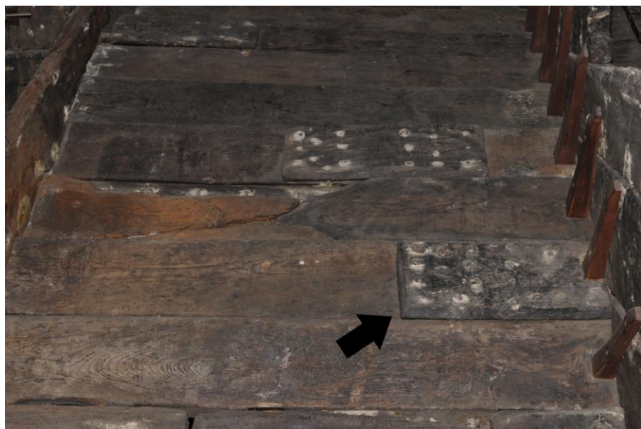
Figure 6-14 Butt strap attached into the bulkhead plank. Photo by author
