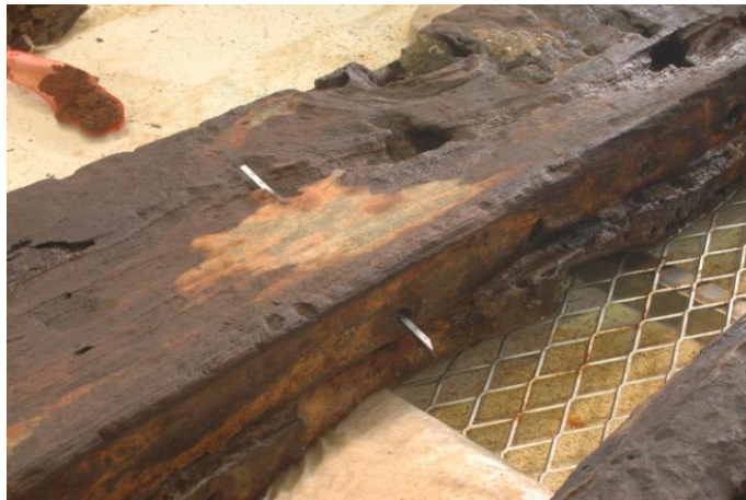
Figure 7-6 Nail that has been diagonally driven from the surface to the lower seam. Photo by author
