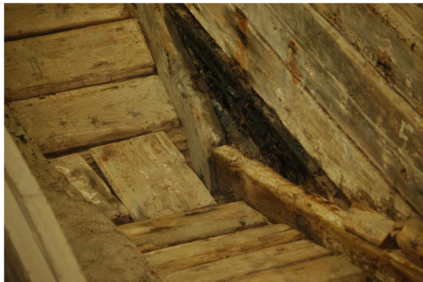
Figure 5-23 Bilge boards (or bottom ceiling planks). Photo by author
