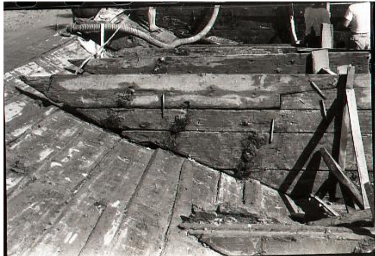
Figure 5-18 Iron clamps fastening bulkheads planks together. Courtesy of Museum of Overseas Communication History
