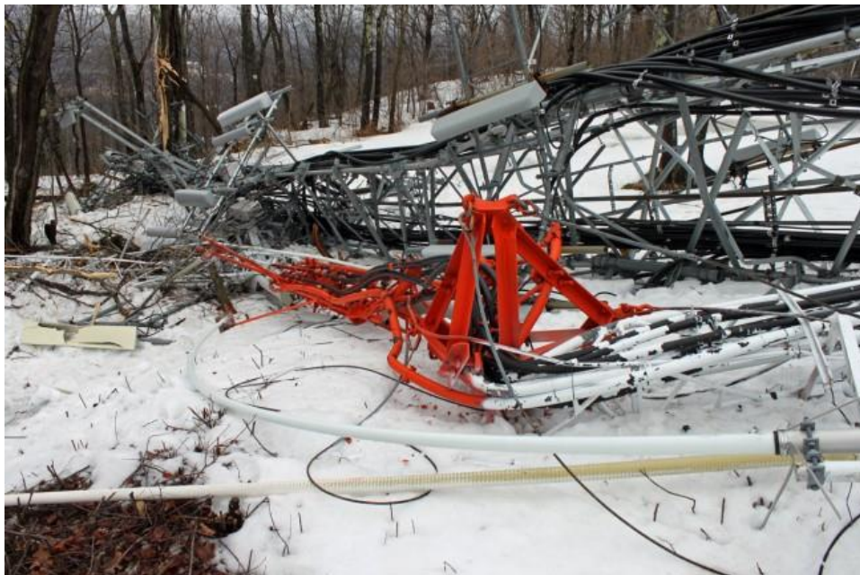
Figure 2. Mobile tower crushed due to natural disaster in North Adams (Thurst 2014)
