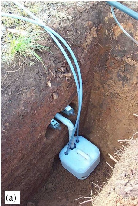
Figure 2.4 Installation of capillary wick lysimeters
