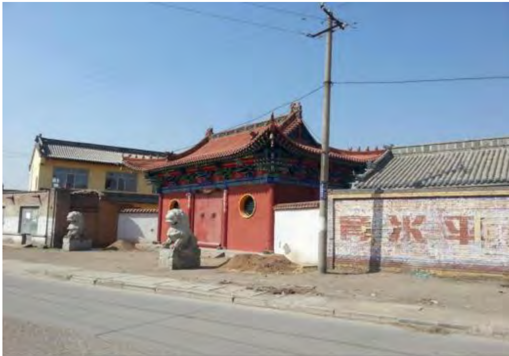
Figure 23. South Temple Gate
