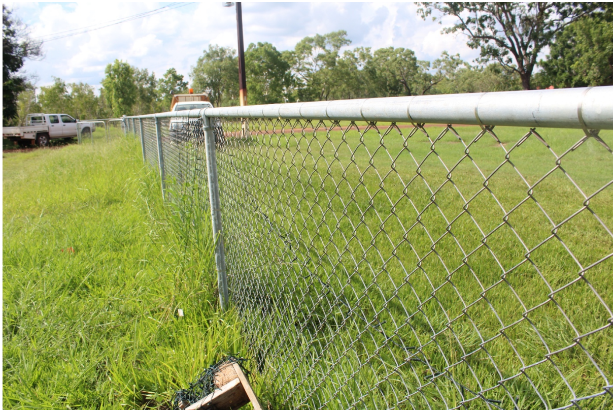
Figure 147. A typical fence in Barunga (Lot 208). This fence is of the newer style of fence built in Barunga (c.2012-2015), as indicated by the presence of the top rail. Photograph by Jordan Ralph, January 2017.
