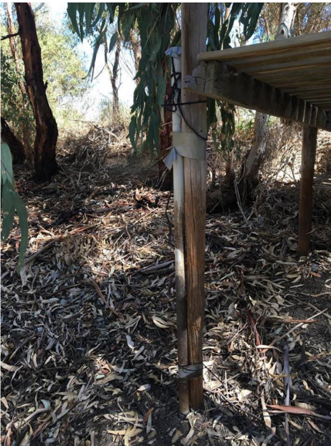
Figure A4: Screening well at the jetty, April, 2018
