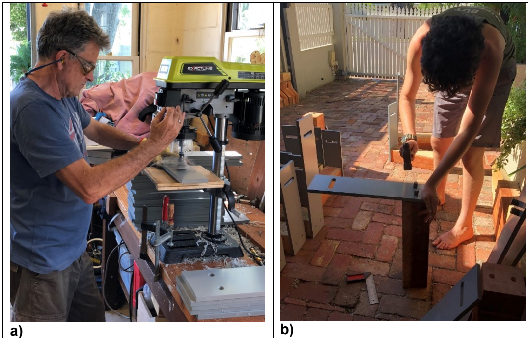
Figure 3.8 Sleeper endplates: (a) fabricating; and (b) assembling (photograph (a) by David Winton, photograph (b) by Trevor Winton).
