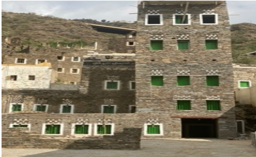
Figure 20: Renovated ancient buildings in Rijal Almaa (Photograph: A. Alfaifi).
