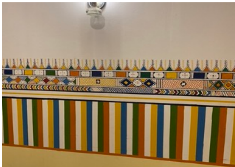
Figure 21: Rijal Almaa's traditional decoration style is applied by women in restoring the ancient buildings' interiors (Photograph: A. Alfaifi).
