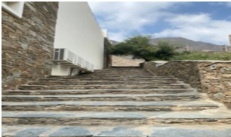
Figure 22: Reconstructed roads in Rijal Almaa, easing access to crucial cultural heritage properties in the village (Photograph: A. Alfaifi).
