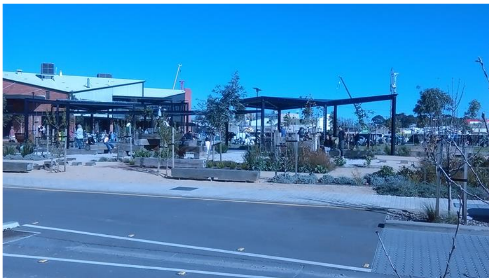
Figure 6.3 Bowden Hub, retail and public open space (from the north)
