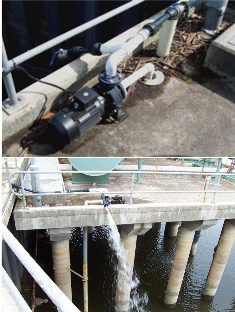
**Plate 3.7.** Installation of the primary pump situated on the weir above the Hope Valley reservoir.
