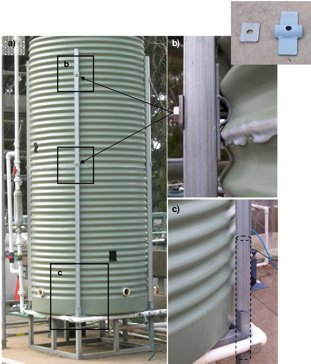
**Plate 3.4.** External media support frame: (a) external posts which support internal media support frames; (b) external mounting bracket; and (c) 1 of 4 external posts positioned over a cylindrical peg.
