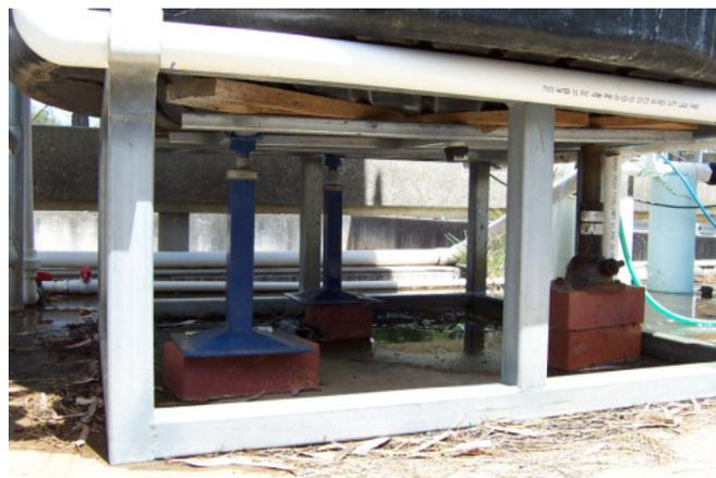
**Plate 3.16.** NTF support stand: Base of NTF column sagging due to excessive accumulation of biomass and the absence of horizontal steel struts. Carjacks were used to help support the base. Car-jacks were later substituted with horizontal support struts (see Section 3.2.2).
