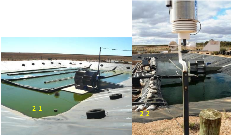
Plate 2-1 & 2-2 Original HRAP configuration (left), modified HRAP configuration and weather station (right)
