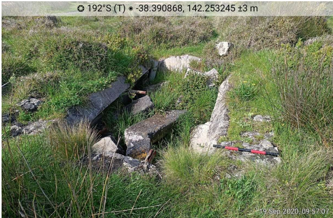
Figure 35: Collapsed bluestone cistern located on the east of Griffiths Island.
