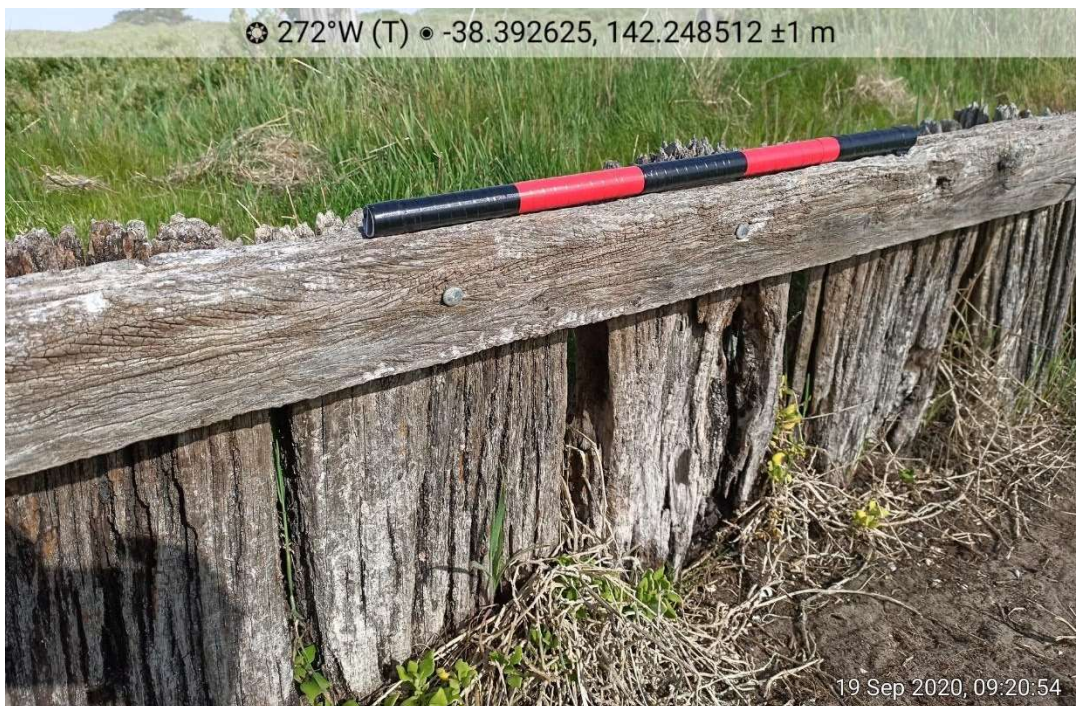
Figure 31: North wall uprights with horizontal bracing (10cm scale divisions).
