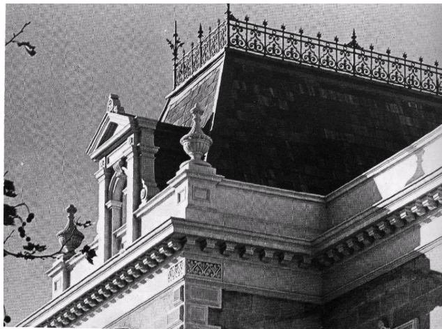
ACC9.1 Mansard roof with cast iron cresting.
