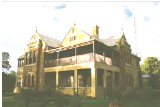
PE 1.7 Bishop's Palace, south west corner. The balcony has been restored; the verandah posts are not original. Photo: R. M. Stone, June, 2009
