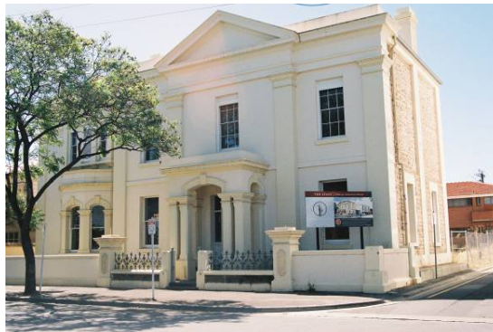
ACC(2) 3.2 Belmont House , street view; engaged columns on the front elevation and random rubble limestone on the east elevation.
