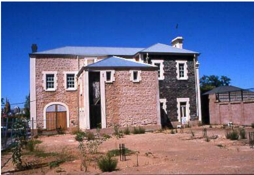
ACC(2) 3.2 Belmont House , rear elevation. The early section on the left is random random rubble limestone construction; the later additions are blue stone. Photo: R. M. Stone, July, 2004
