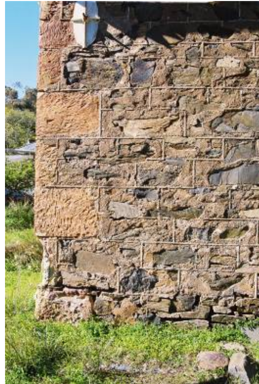
LI5.4 Yatara , squared stone quoins and random rubble construction of the early cottage. N100.
