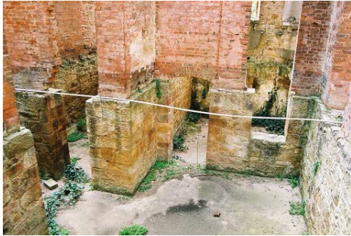
AH8.8 Marble Hill , the cellar; ashlar construction. Photo: R M Stone, September, 2007
