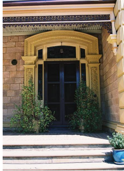
ACC(2) 26.4 Strellda , front entrance. N165. Ashlar limestone construction. Photo: R. M. Stone, November, 2007
