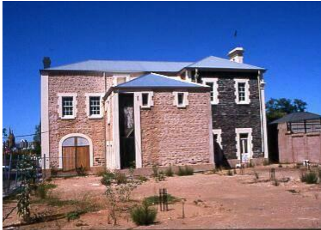
Figure 5.28 Belmont House . Left: the first stage built of limestone with random rubble construction. Right, the second stage built of squared bluestone. Photo: R. M. Stone, July, 2004
