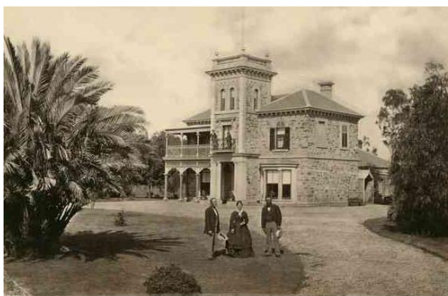
Figure 6.7 The Brocas , c1876, with later additions, including, the tower, verandah and balcony. The original cottage can be seen in the rear. Source: SLSA, B 10656.
