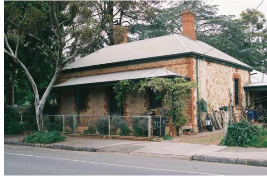
Figure 2.4 Free standing cottage, Albert Street, Mitcham, (Mitcham Conservation Zone), c1870s.
