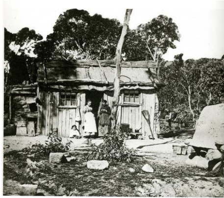
Figure 5.1 Country cottage with vertical sawn board walls and a bark roof kept flat by saplings. Source: O'Neil, 1982:16.
