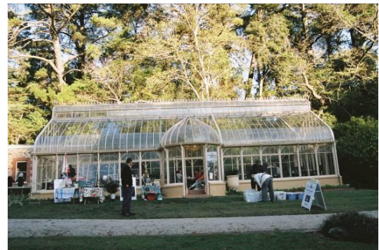
Figure 7.22 Beechwood . The former Birksgate conservatory, now an entertainment area. N180. Photo: R. M. Stone, May, 2009.
