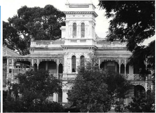
Figure 5.25 Eynesbury , c1982. Elaborate lace balustrades on the balcony; lace friezes and brackets on both the verandah and balcony.
