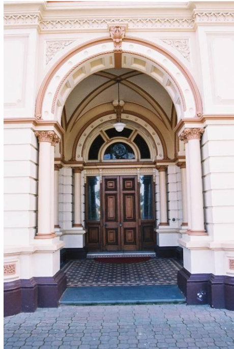
Figure 5.41 Paringa Hall . Main entrance with columns, elaborate plaster and stained glass Photo: R. M. Stone, September, 2007
