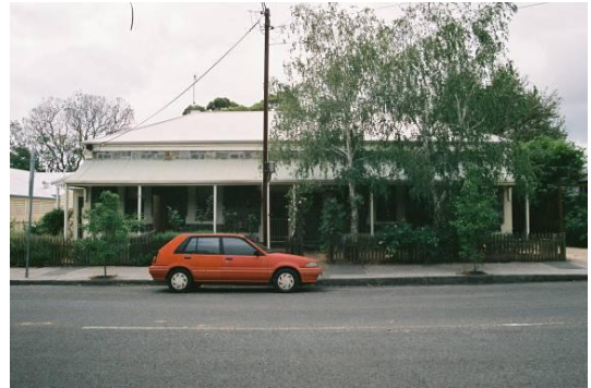
Figure 2.2 Workers' Cottages, Loch-Ness Avenue, Torrens Park (Mitcham Conservation Zone), c1870s. Photo: R. M. Stone, December, 2009
