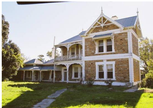
Figure 5.5 Yatara : the early cottage is on the left. Note: the wooden balcony balustrade and wooden friezes. Photo: R. M. Stone. July, 2007
