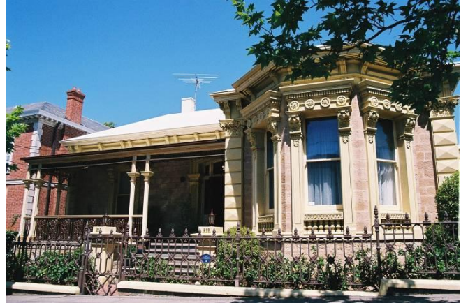
Figure 5.32 Strelida , North Adelaide decorative quoins and plaster mouldings. Photo: R. M. Stone, November, 2007
