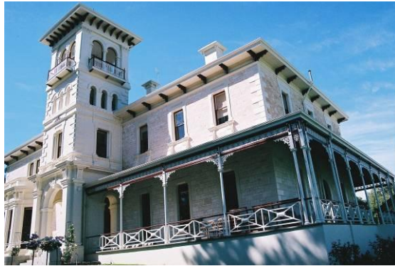
Figure 5.24 Struan House , No balcony; verandah with lace brackets.
