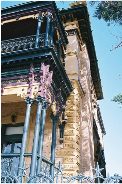
Figure 5.31 Albert Hall , Glenelg: decorative quoins and associated moulded plaster work. Photo: R. M. Stone., June, 2006
