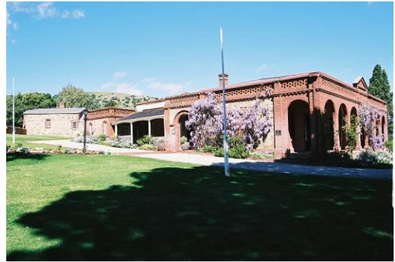
Figure 6.11 Beaumont House ; arcade verandah on the right and main entrance now on the left (north elevation). Photo: R. M. Stone, September, 2006
