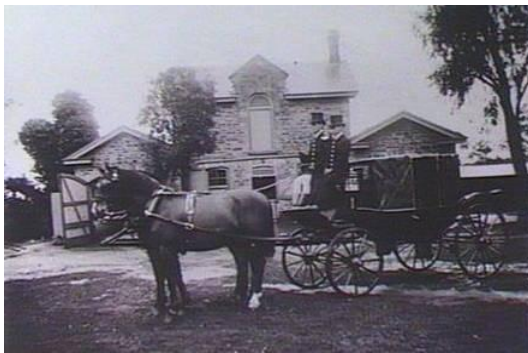
Figure 7.13 Benacre coach house and stables, c1906 Coach house doors on left.
