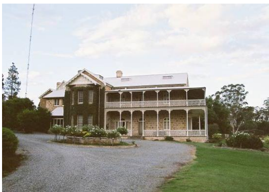
Figure 5.9 Bungaree : an asymmetrical house with bay windows on the left, verandah and balconies on two sides, both with lace balustrades. Photo: R. M. Stone, March, 2007
