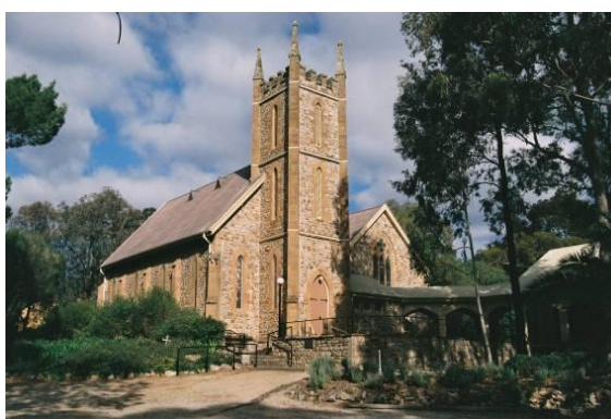
Figure 4.10 St Michael's Anglican Church, Mitcham. Photo: R. M. Stone, December, 2009.
