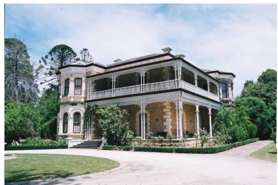
Figure 5.10 Yallum Park : an asymmetrical design with a faceted bay windows, verandahs and balconies on two sides with lace balustrades on the balcony. Photo: R. M. Stone, November, 2007
