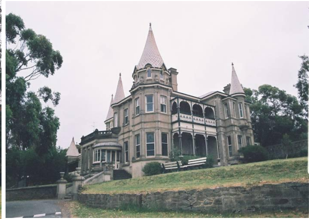
Figure 5.40 Adare , Victor Harbor: elaborate turrets with ‘candle snuffer’ roofs. Left: garden stairs provide an entry and exit to the ballroom
