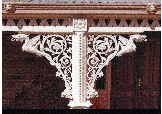
Figure 3.5 Dalintober , cast iron verandah brackets with dragons. Source: Raine & Horne sale brochure, 2009
