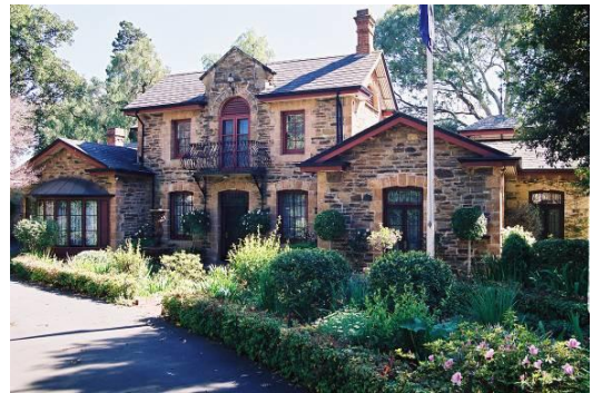
Figure 7.14 Benacre coach house and stables. Coach doors converted to a bay window. Balcony added to loft doorway.
