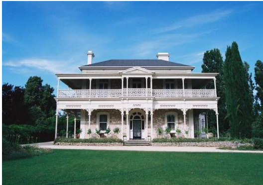
Figure 5.26 Padthaway , in the southern country region, lace balustrades brackets and friezes decorate all sides. Note: there is no balustrade on the verandah. Photo: R. M. Stone, November, 2007
