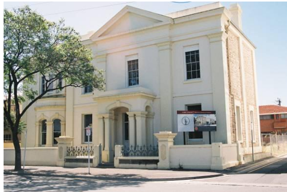
Figure 5.21 Belmont House . Plastered front elevation with engaged columns and portico entrance.
