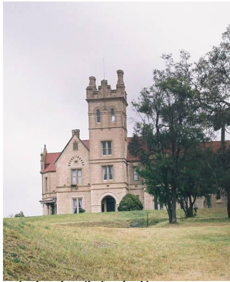
protruding above the four level tower.
