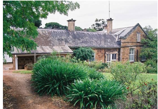
Figure 5.8 Hill River Station : on the left the early section of the house: note the original slate roof and house and intersection with the later additions. Photo: R. M. Stone, March, 2007
