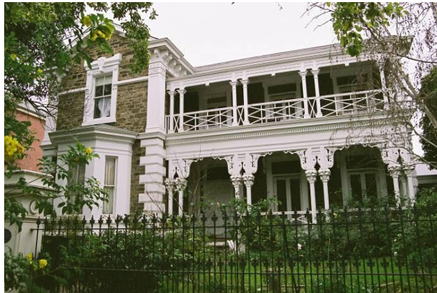
Figure 5.22 Parramatta Villa , North Adelaide. Elaborately carved timber verandah posts capitals and brackets. Photo: R. M. Stone, November, 2007
