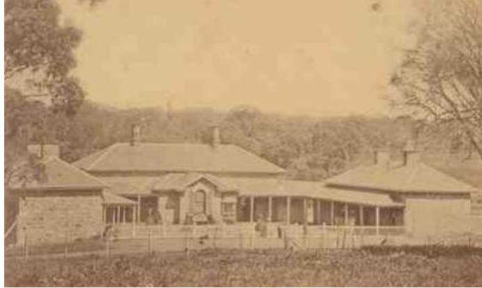
Figure 6.3 Anlaby , c1860. Family quarters on the left, kitchen and servants' quarters on the right. Source: SLSA, B 21351
