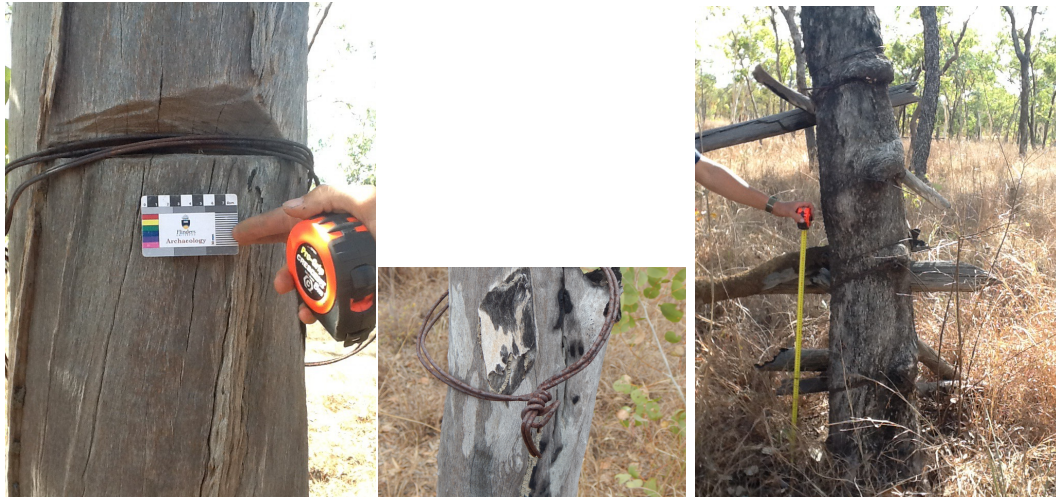
Figure 77: Left: Image of a typical post at Clayhole Yards 1 showing horizontal mark is only wide enough to support the wire for the horizontal rails. Centre: shows a Cobb and Co knot at Clayhole 1. Right: shows tree used as yard post with horizontal rails attached with wire through tension (tape is 1m in length).
