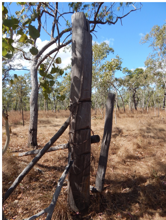
Figure 75: Entry post at Clayhole Yards 1, to the left of the main post are some horizontal rails still attached.
