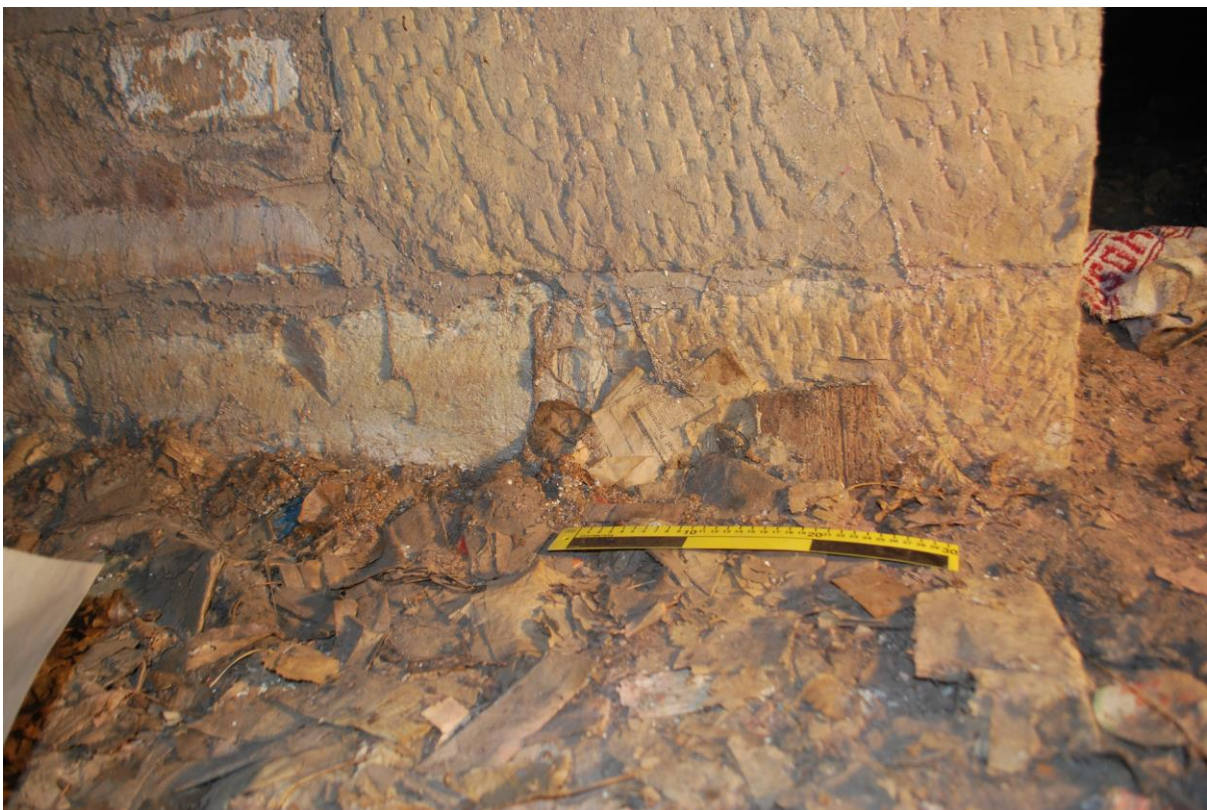
Figure 74: Underfloor space Ladies' Cottage. Photograph by Lynley Wallis, February 2017.
