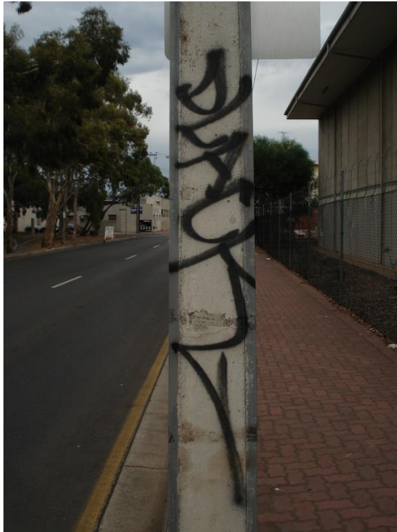
Figure 3.2. Stobie pole, City of Charles Sturt
