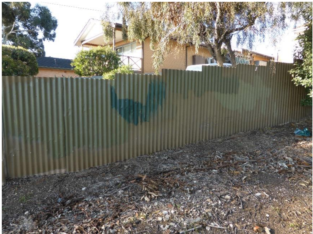
Figure 3.4. Removed graffiti, Ocean Boulevard, City of Marion
