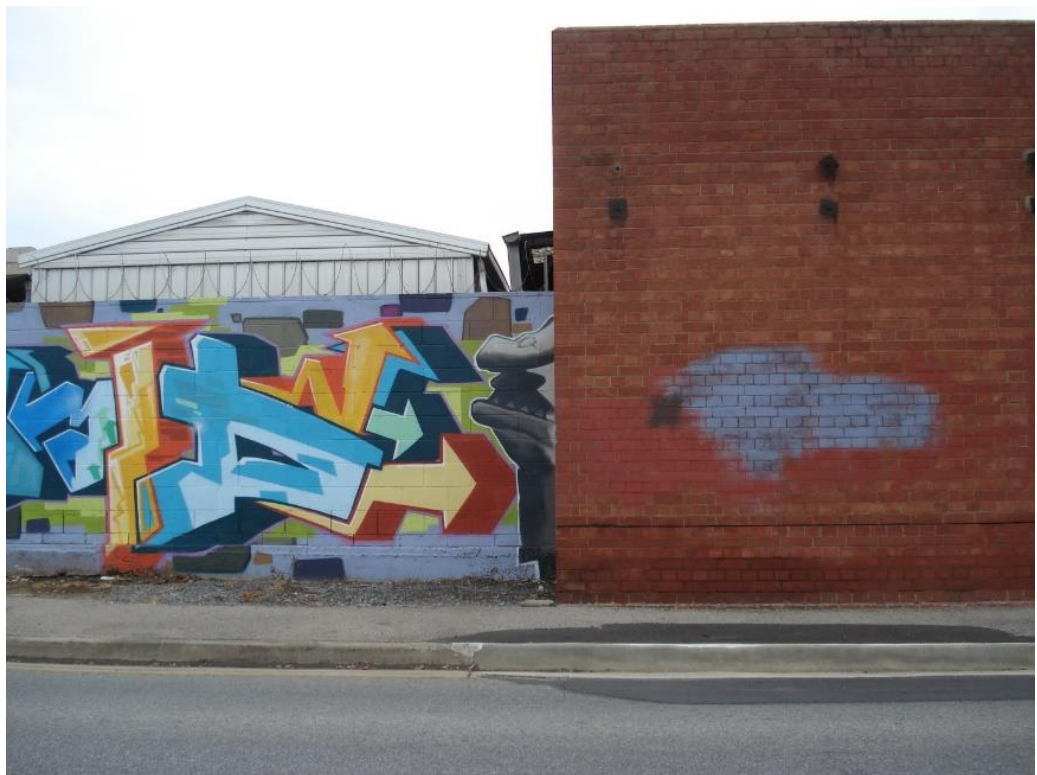
Figure 4.2. A graffiti piece and a paint smudge, City of Charles Sturt
