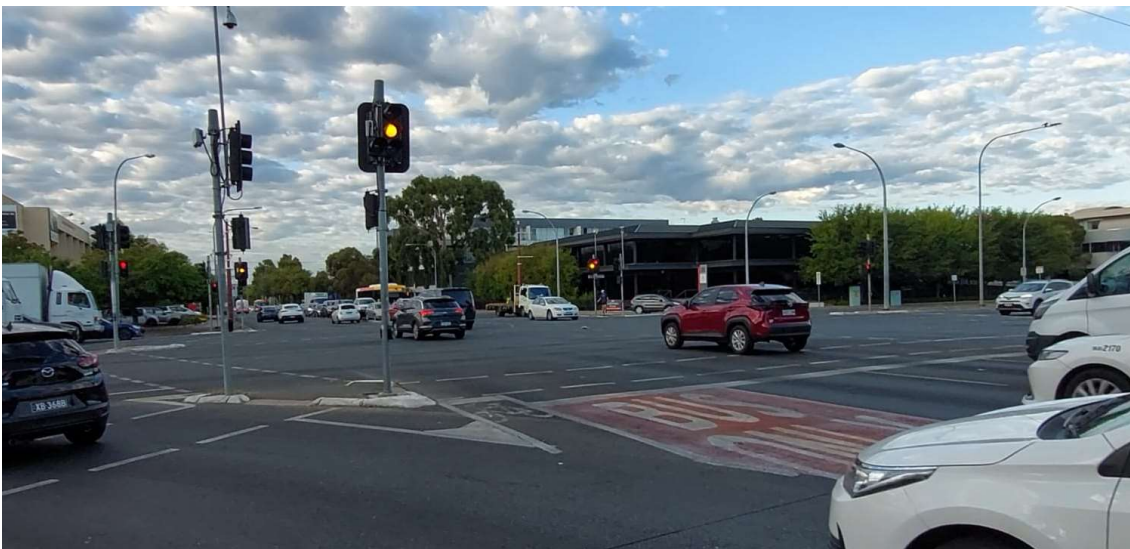
Figure 4: Site Survey on Goodwood Rd
