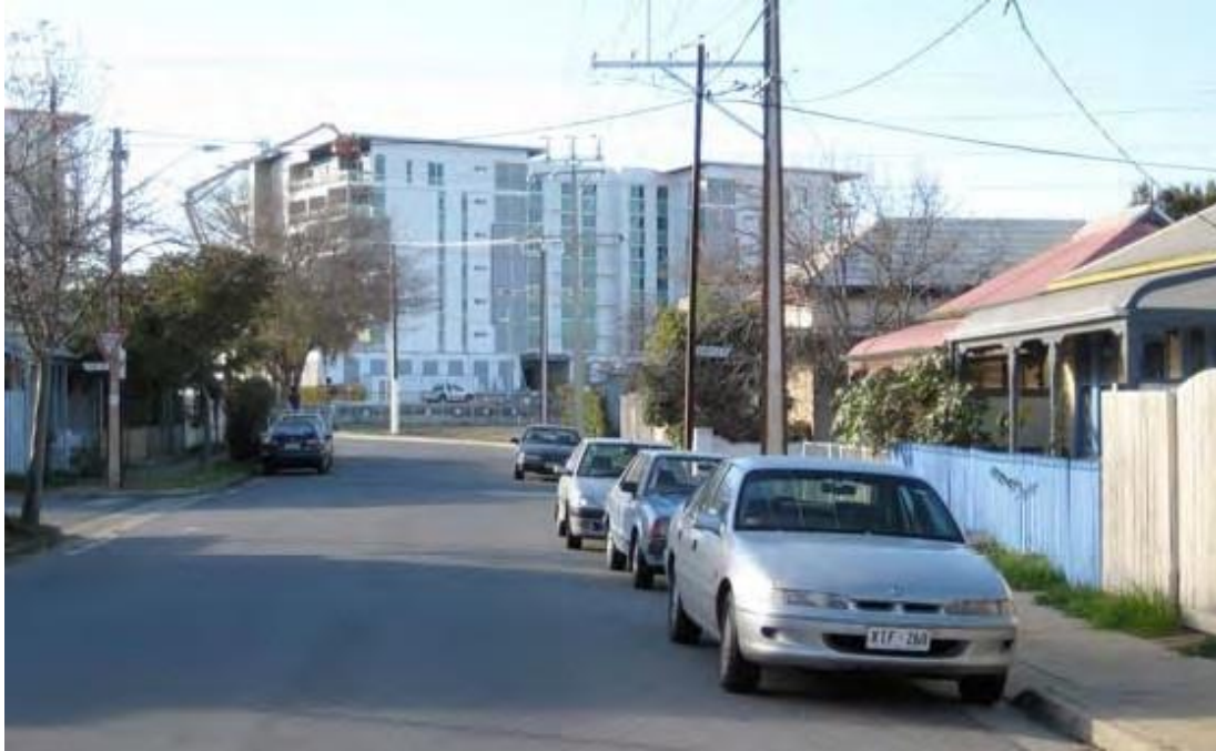
Figure 11: View of seven storey Stage 2A buildings, illustrating the sharp contrast between Newport Quays and the surrounding suburbs (photograph T. Kearney).
