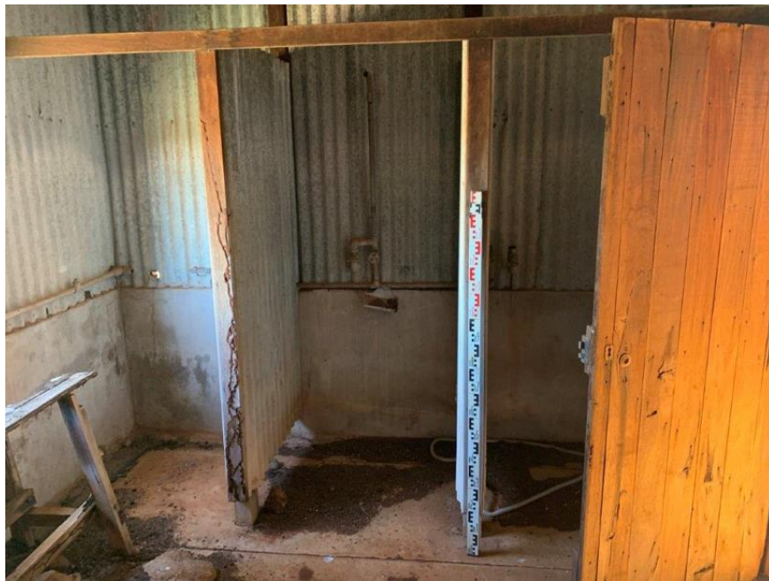
Figure 32: Timber in shower room of shearers' quarters. (Photograph: Bart King)
