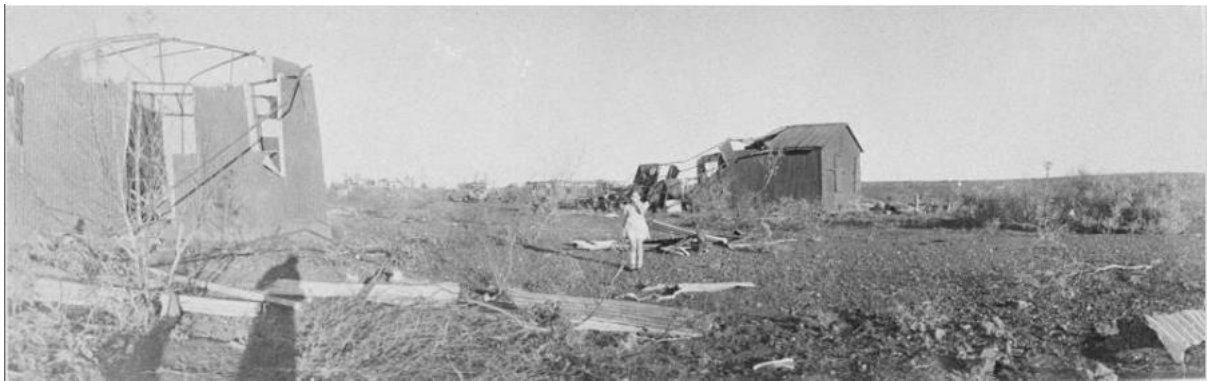
Figure 5: Balmoral Station shearers' quarters and dining room after 1945 cyclone. All structures in photograph demolished after cyclone.
