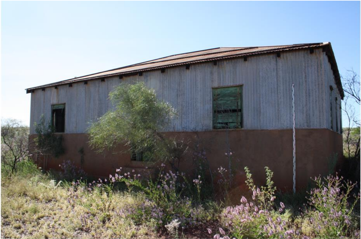
Figure 24: Balmoral dining hall western side. 1.6m concrete wall. (Photograph: Bart King)
