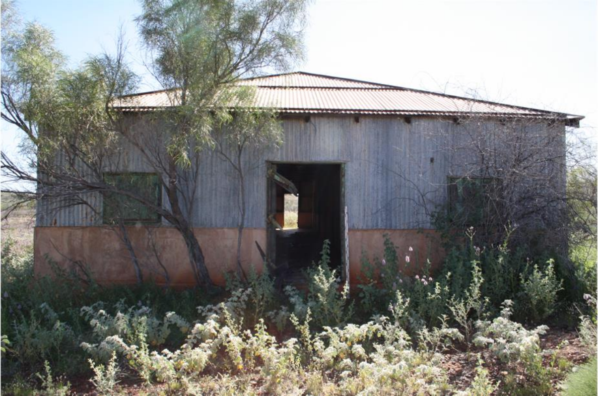
Figure 26: Balmoral shearers' quarters southern end. (Photograph: Bart King)
