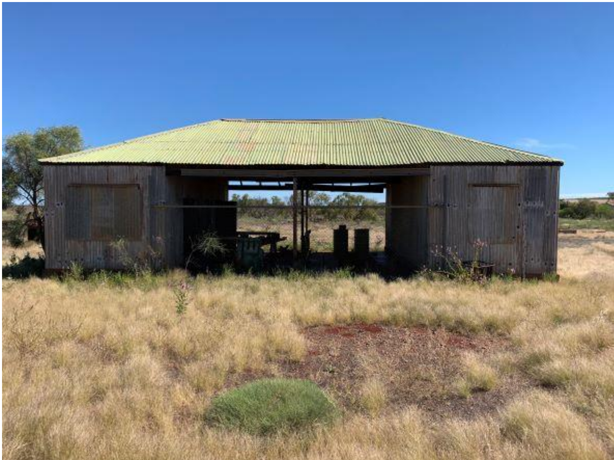
Figure 34: Balmoral precinct workshop building. (Photograph: Bart King)
