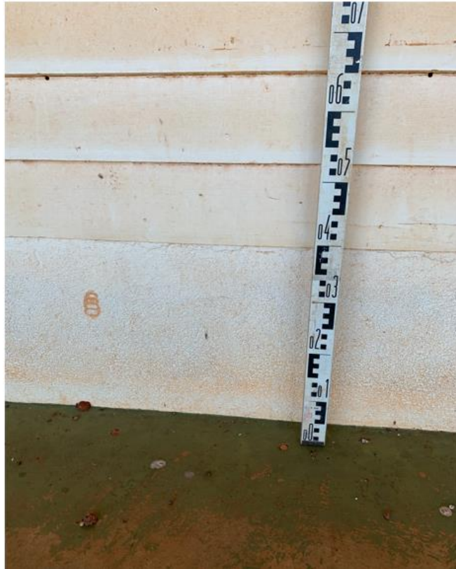
Figure 16: Height of concrete walls at Balmoral homestead (Photograph: Bart King).
