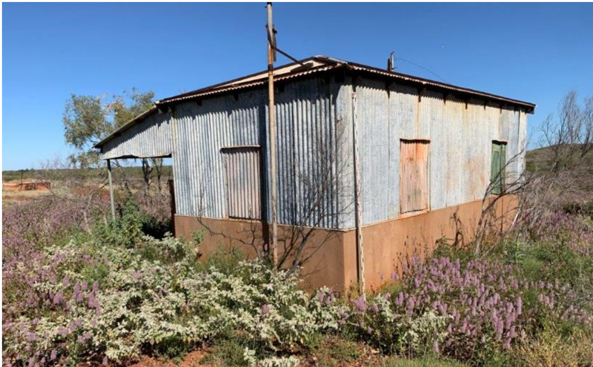
Figure 19: Balmoral supervisor's building showing hipped roof and window shutters. (Photograph: Bart King)
