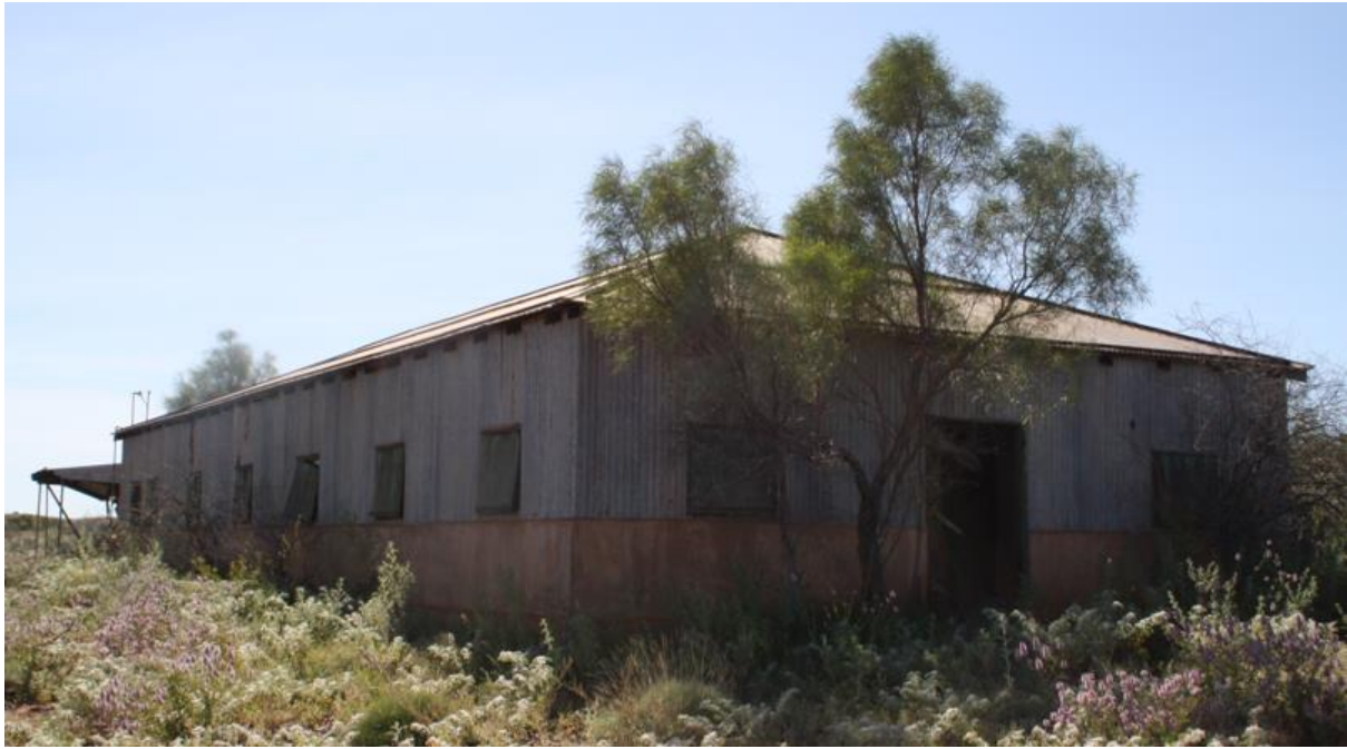
Figure 28: Shearers' quarters roof design (Photograph: Bart King)
