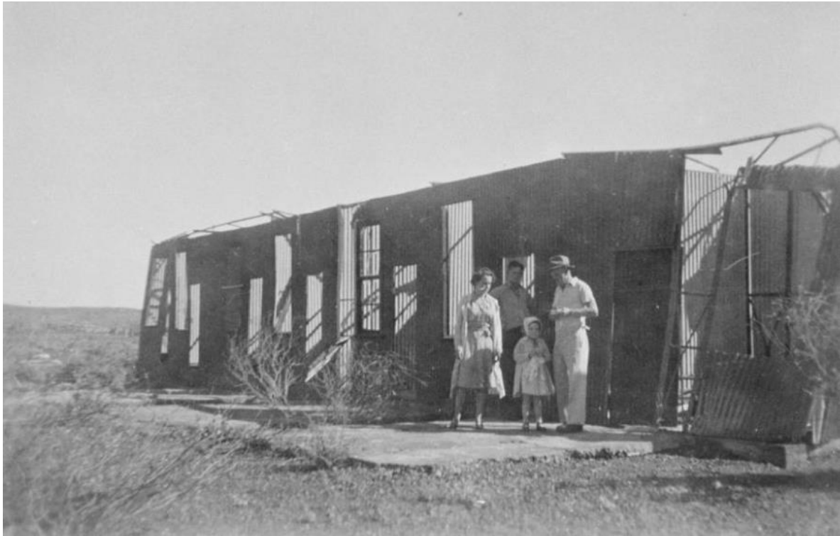
Figure 6: Balmoral shearers' quarters after 1945 cyclone.
