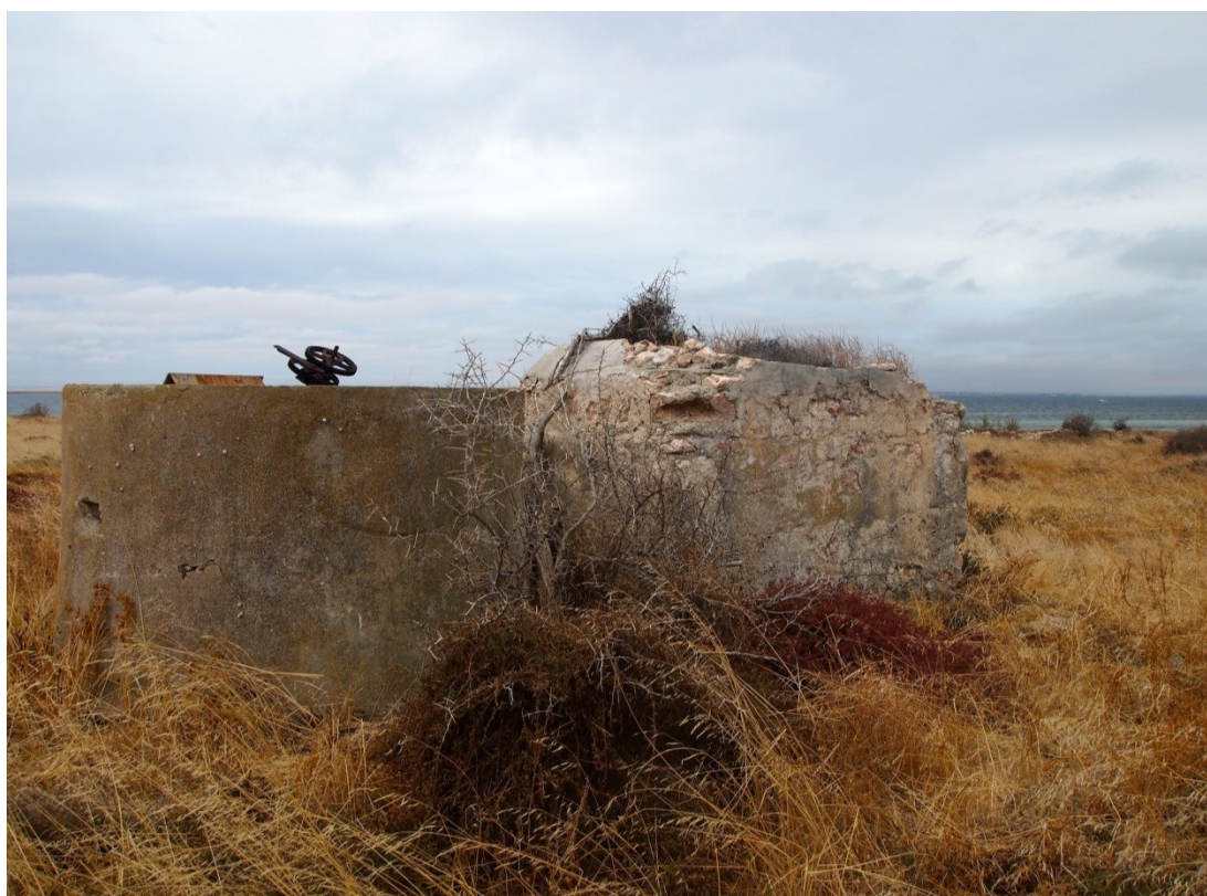
Figure 103 Tank Stand 1 showing the square and circular tank with cogs visible, facing northeast towards the sea. The windmill base is behind these tanks (photograph by A. Roberts 25/2/13).
