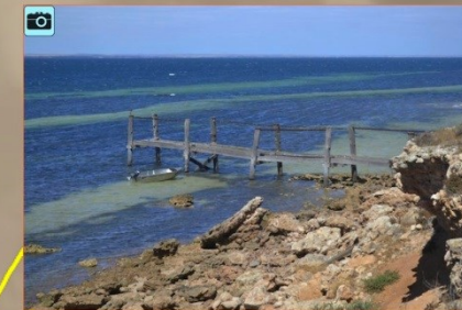
Replica of the above photo – note that some of the metal rails along the top, the diagonal timbers at the end of the jetty, and all the planking on the jetty is no longer there (28 February 2013 M. Fowler).
