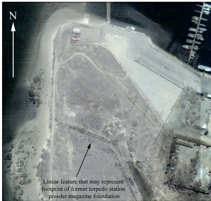
Figure 3. Aerial photograph of North Arm Torpedo Station, ca. 1961, overlaid on an aerial photograph of the modern landscape. Of particular interest is a linear feature that may represent a portion of the former torpedo station magazine foundation. Archival photograph courtesy Jan Perry Private Collection; modern aerial image courtesy Google Earth.
