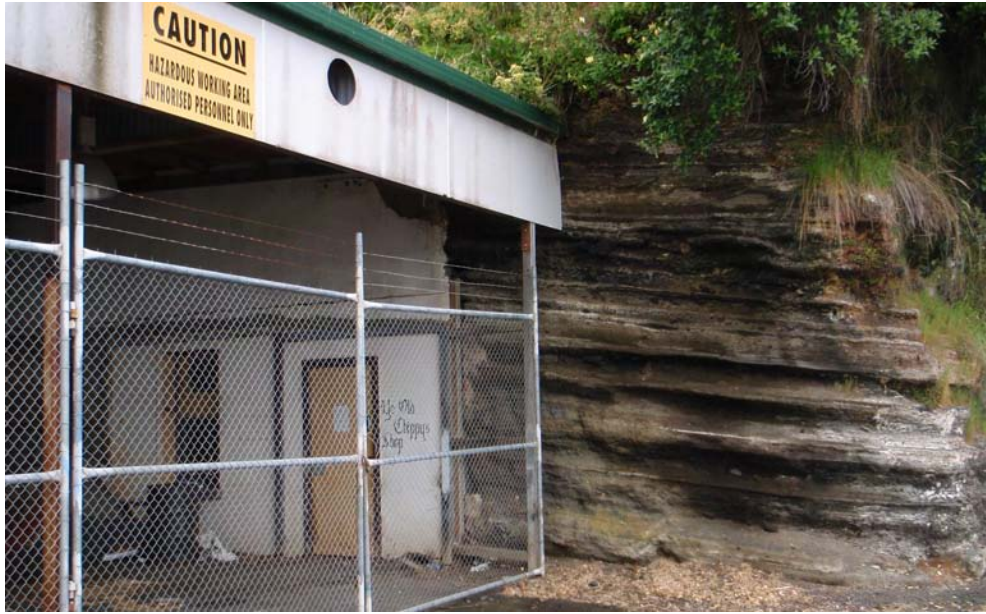
Figure 30. The Torpedo Bay station's former test room, as it appeared in November 2008. This subterranean structure was built into the cliff face and originally used to test torpedo detonators and other explosive devices. Entrance to the test room was through the yellow door just inside the fenced enclosure.
