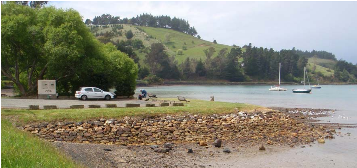
Figure 46. The Deborah Bay Submarine Mining Station mole, as it appeared in November 2008. Note the structure's robust stone and earthen construction, as well as its current use as a car park (signage describing the mole's historic role as an element of the submarine mining station is located immediately to the left of the white car).
