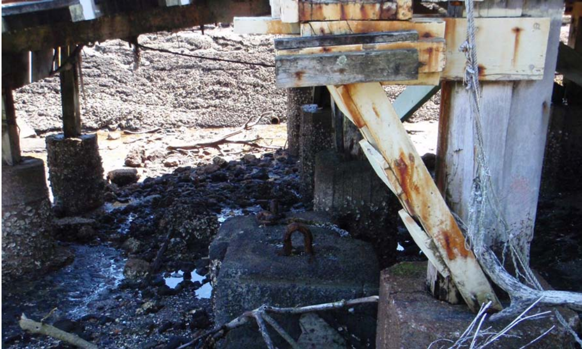
Figure 33. Underside of the Torpedo Bay Submarine Mining Station's extant slipway as it appeared in November 2008, showing deteriorated and damaged wooden pile (in centre of image). Note extensive iron staining on structural supports in foreground, as well as accumulated debris and rubbish.
