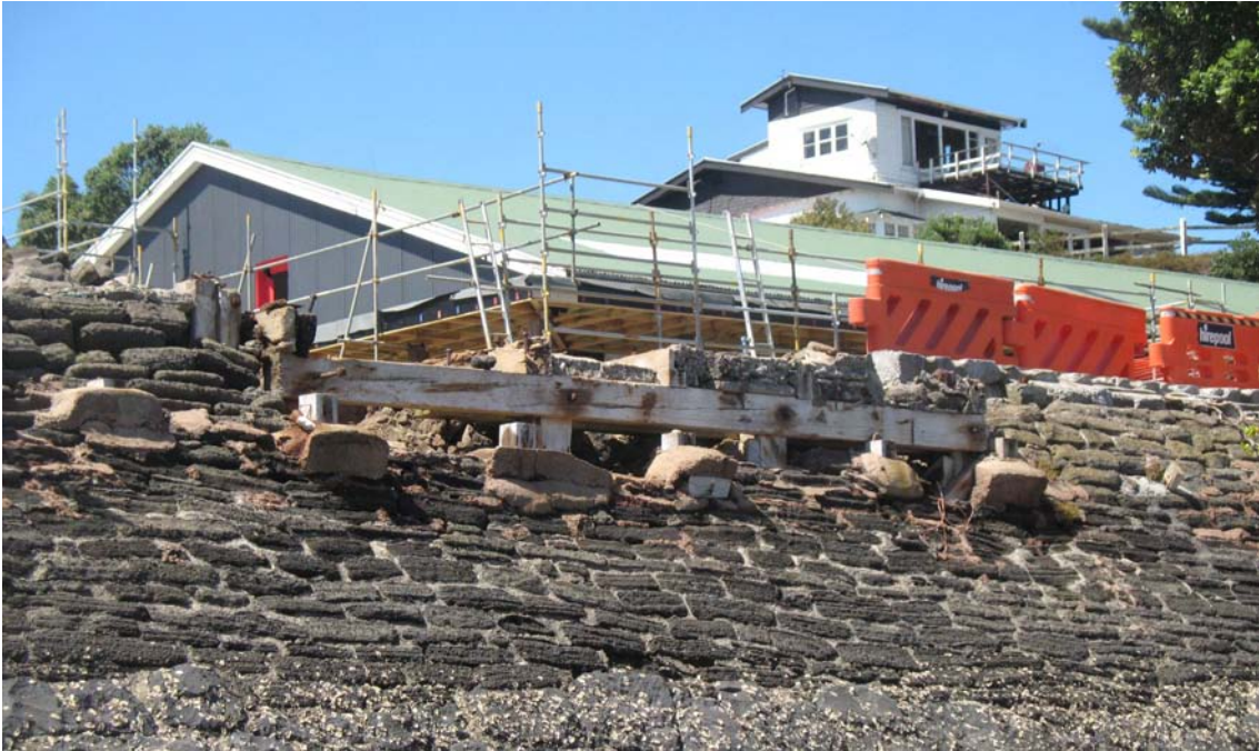
Figure 28. Remnants of the Torpedo Bay Submarine Mining Station's 1886 wooden jetty head, as exposed during archaeological investigations in 2009. Image courtesy of Opus International Heritage Consultants.
