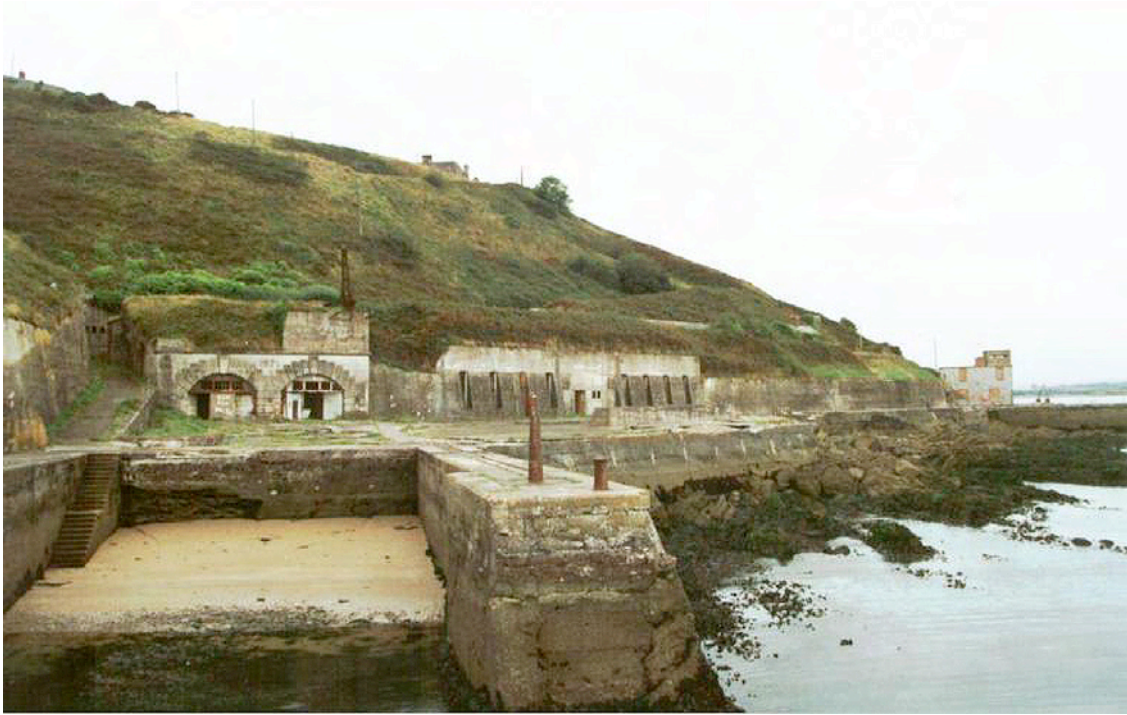
Figure 83. The submarine mining establishment at Fort Camden (Cork, Republic of Ireland), showing its stone and masonry buildings, boat basin, and dock infrastructure. Image courtesy of the Palmerston Forts Society.
