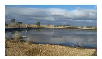
Figure 2.18 – Anaerobic pond upstream Peterborough HRAP
