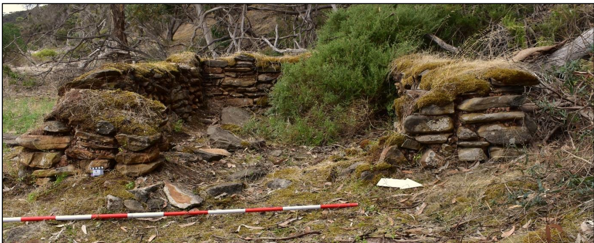
Figure 32: Eastern wall of structure D.
