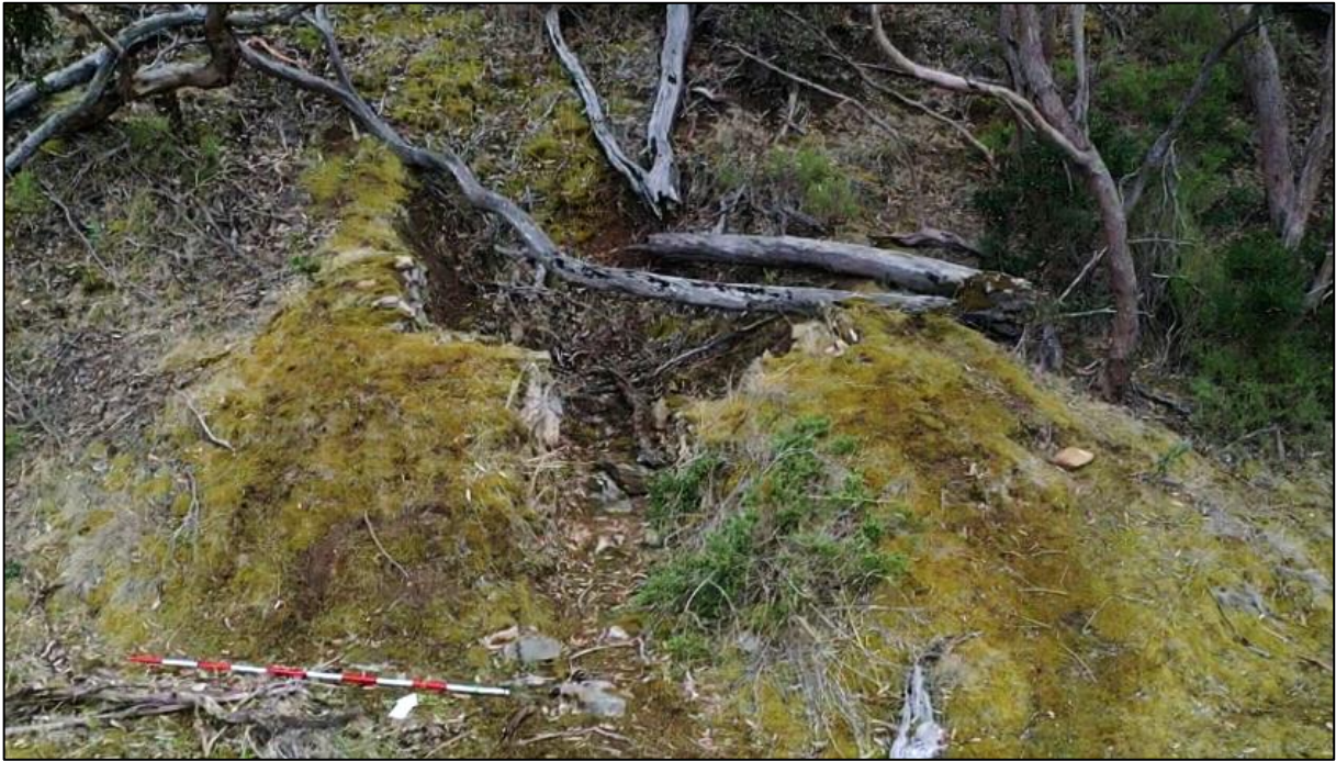
Figure 25: Photo of southern wall of Structure D.
