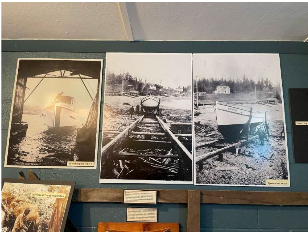
Figure 32 Black and white photographs of vessel repair. (C. Wilkey 2023).
