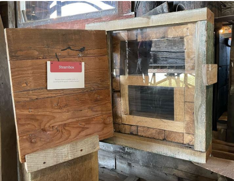
Figure 4 Closeup of the steam box and its attached signage. (C. Wilkey 2023).
