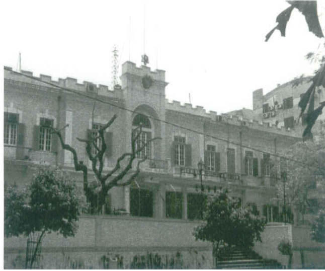
Fig. 20 Traffic Police Headquarters Avenida Sídonia País
