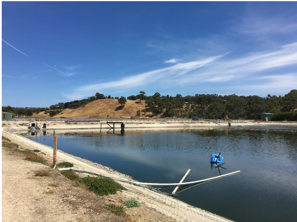
Plate 3.1 Wastewater pumped from the last pond of waste stabilisation pond series
