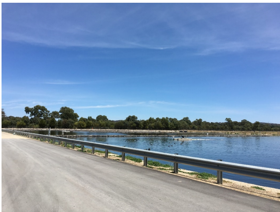
Plate 2.1 Mt Barker Wastewater Treatment Plant, South Australia
