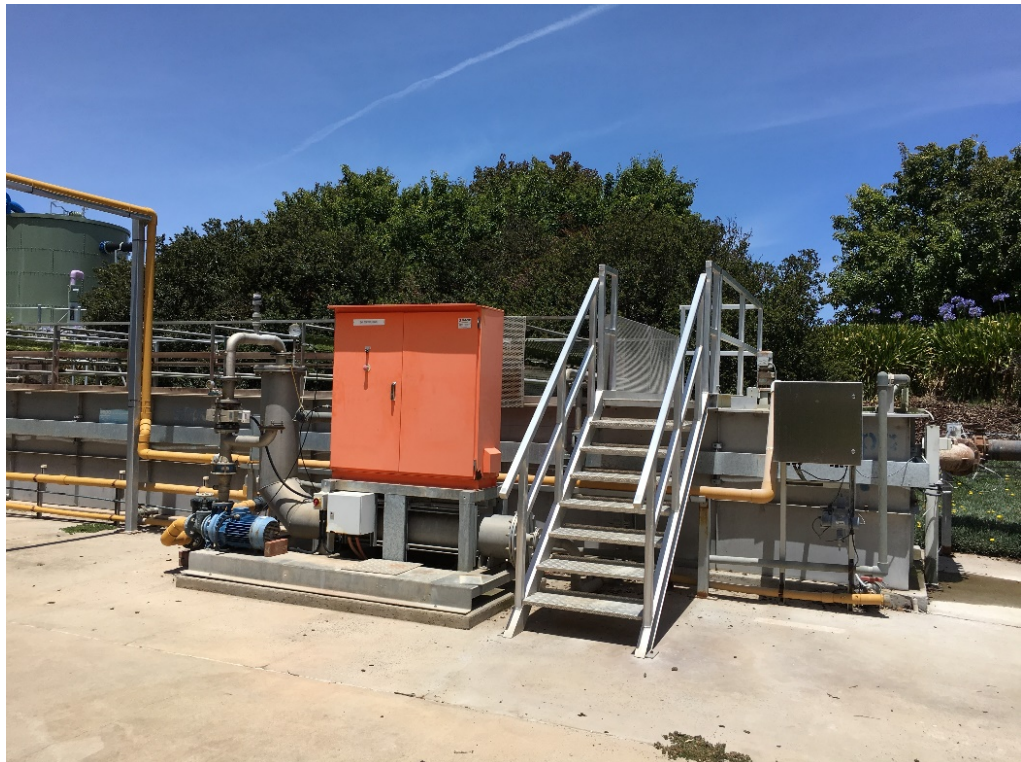
Plate 4.2 Dissolved Air Flotation
