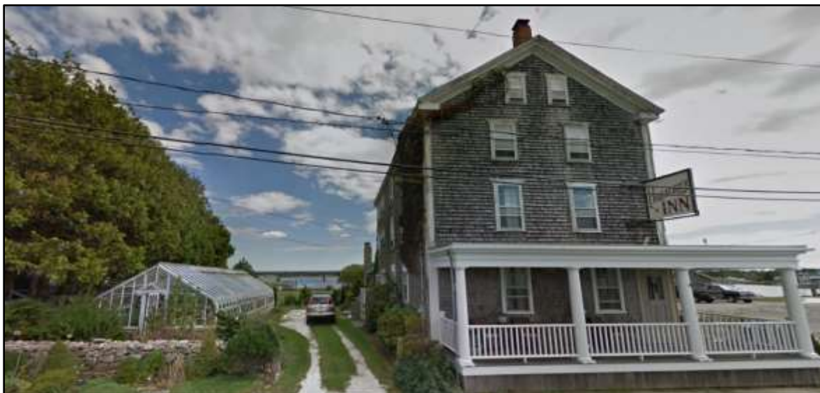
Figure 60. Paquachuck Inn (Cory Store) (right) and former oil storage lot (left) (Google satellite).
