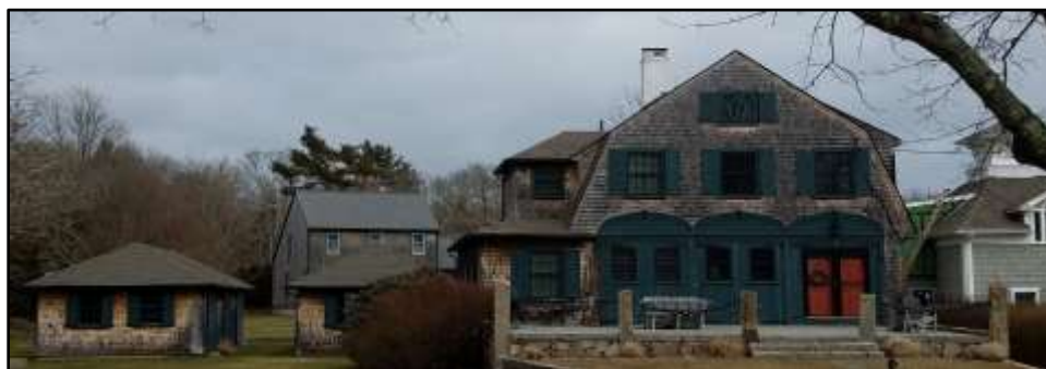
Figure 66. Hall Blacksmith Shop (Photo by author).
