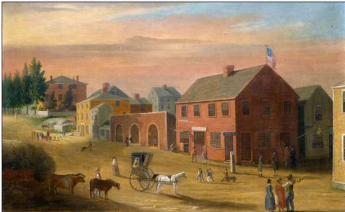
Figure 10. Painting of Water and Williams streets, 1805 (Northwest) (William Wall, 1807).
