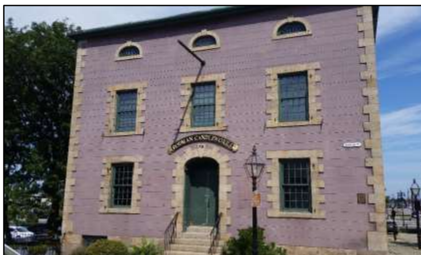
Figure 42. Rodman Candleworks (facing northeast) (Photo by author).
