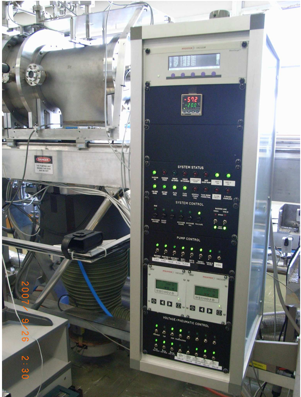
Figure 2.1.7: A photograph of the programmable logic controller and the Pfeiffer Maxigauge pressure monitoring controller, turbo controllers and temperature readout.
