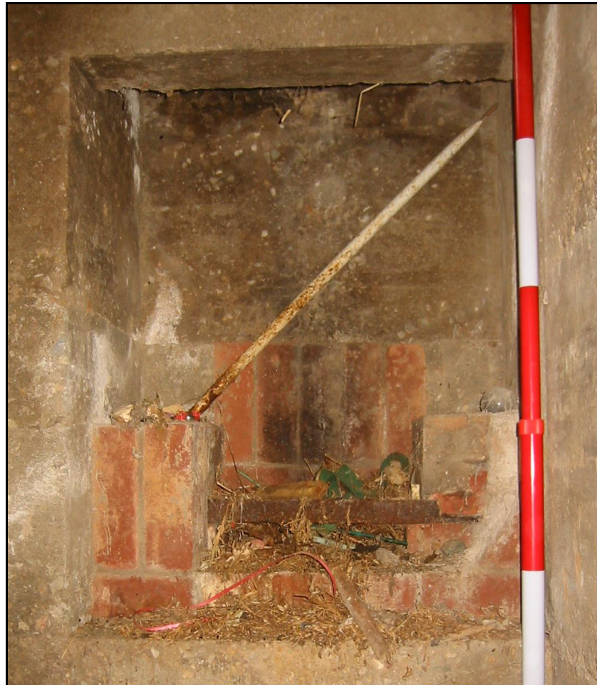
Figure 7-52: Fire place in Willis Type V shelter (Wimmer 2010)
