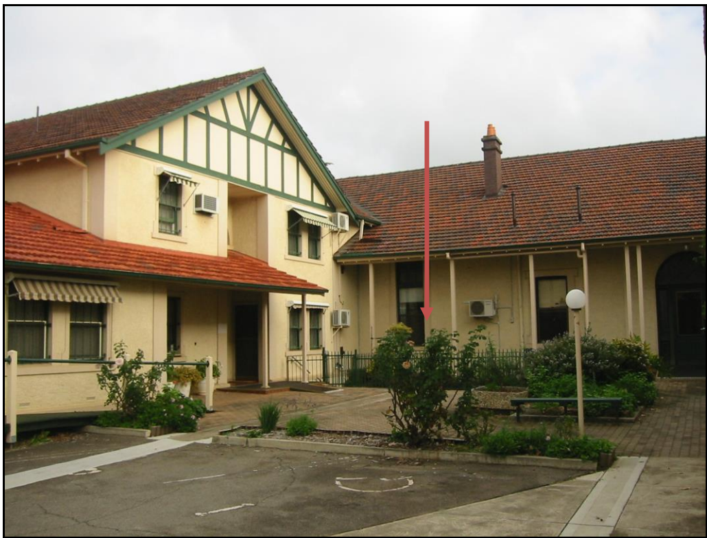
Figure 7-55: Rear of Harley home. Fenced Type V shelter location arrowed (Wimmer 2013)
