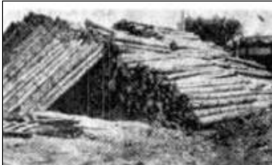
Figure 7-11: Commercial Case Company's Type II shelter ( News , 27 February 1942: 3)
