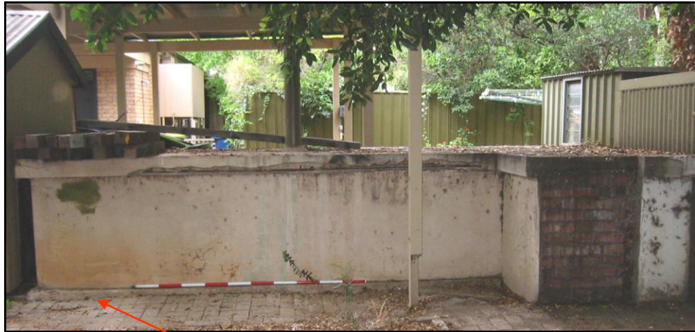
Figure 7-45: External wall thickening evident below range pole in Griff Type V shelter (Wimmer 2008)
