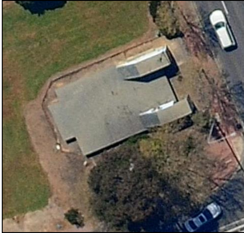
Figure 7-27: Aerial view of Thebarton ARP Sub-Control Station 2010 (URL image www.nearmap.com )
