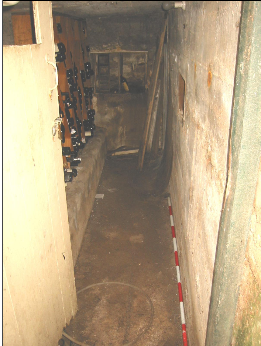
Figure 7-47: Pierce Type V shelter showing concrete bench and built in shelves (Wimmer 2009)
