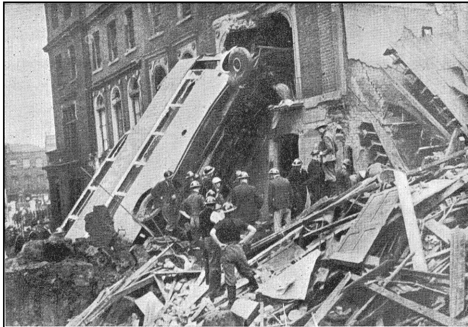
Figure 3-2: Double-decker bus blown into a private residence in London (Browne 1941: 35)
