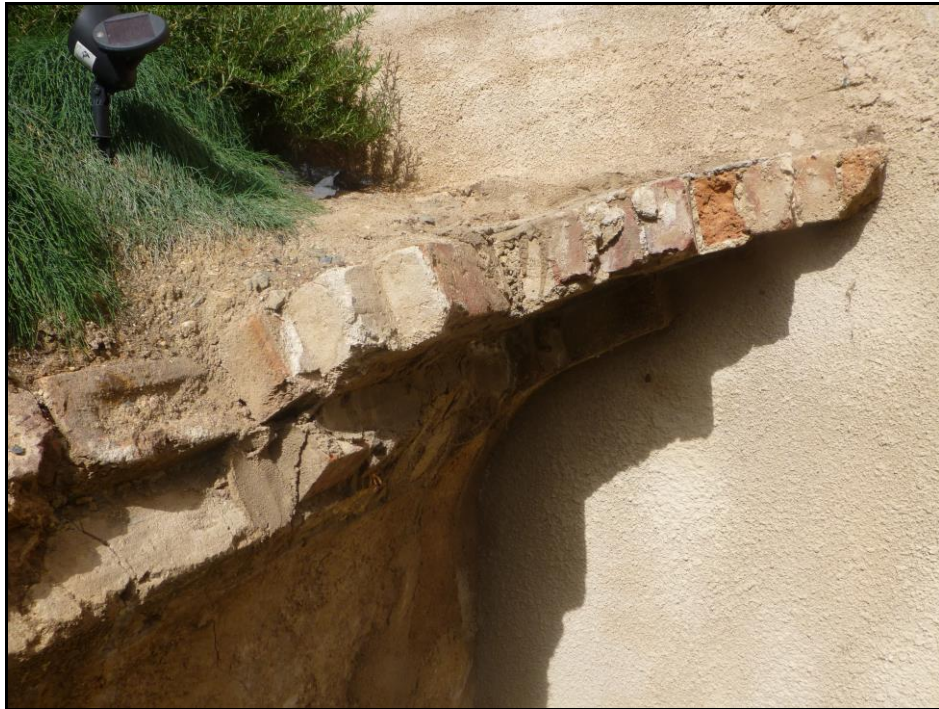
Figure 7-57: Detail of roof vault showing two courses of bricks, Harley Type V shelter (Wimmer 2013)
