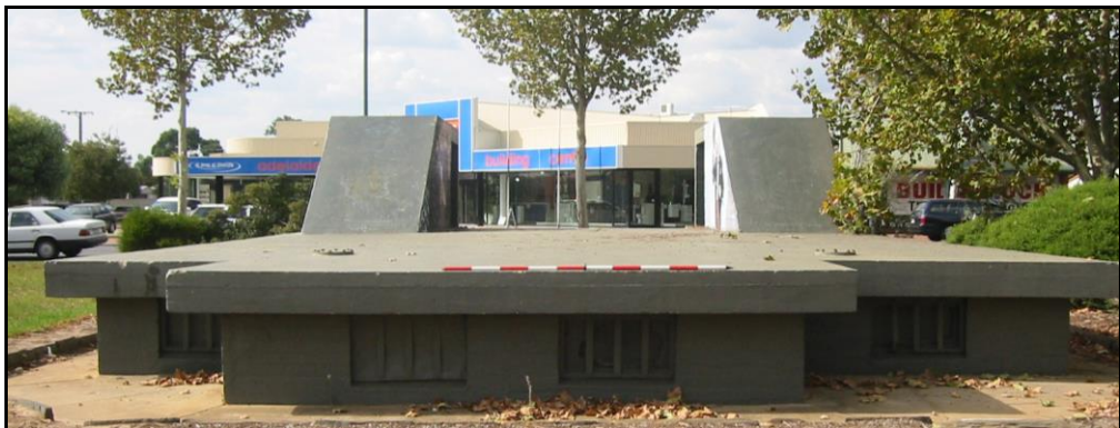
Figure 7-28: Rear of Thebarton Sub-Control Station showing roof overhang (Wimmer 2006)
