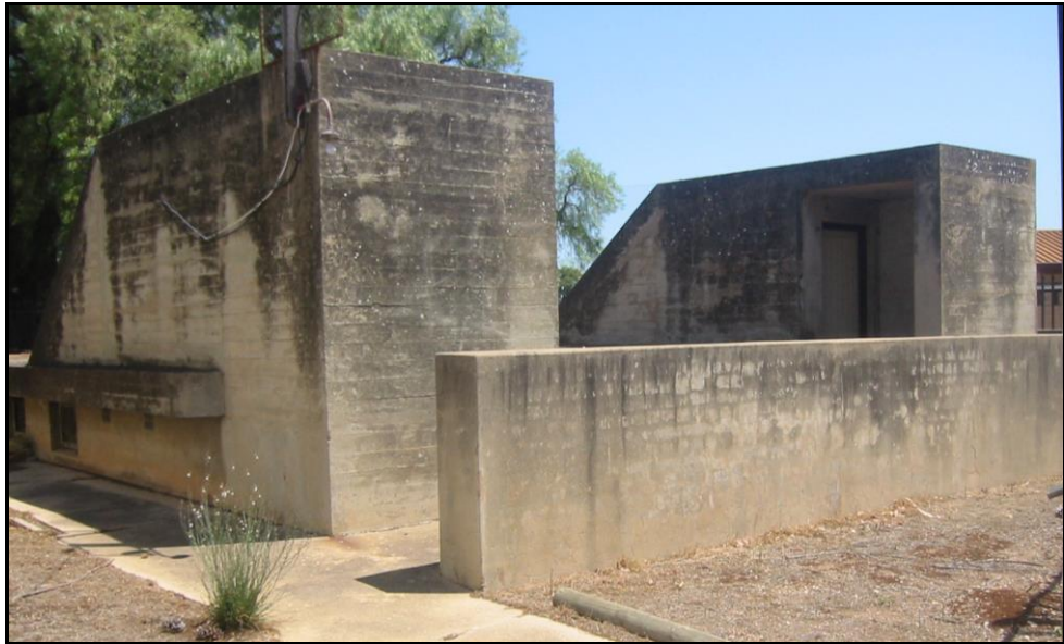
Figure 7-31: Prospect ARP Sub-Control Station showing blast wall across both exits (Wimmer 2007)
