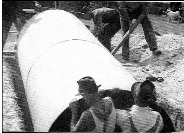
Figure 6-10: Installing a plywood pipe shelter in suburban Sydney, December 1941 (In Fallows 2005: 132)
