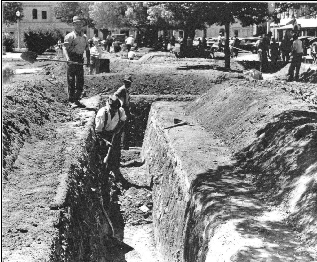
Figure 7-2: Depth of trenches in Victoria Square, Adelaide c1942 (c/o Ray Hirst, NEWS LTD)
