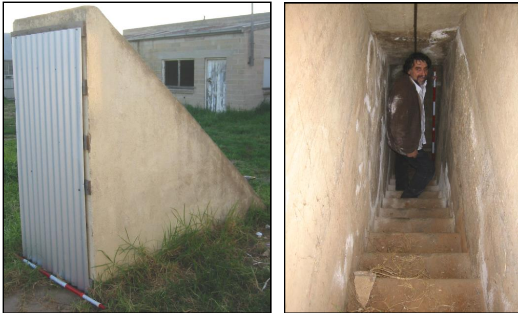
Figure 7-50: Garden exit and steps, Willis Type V shelter (Martin Wimmer and Louise Holt 2010)
