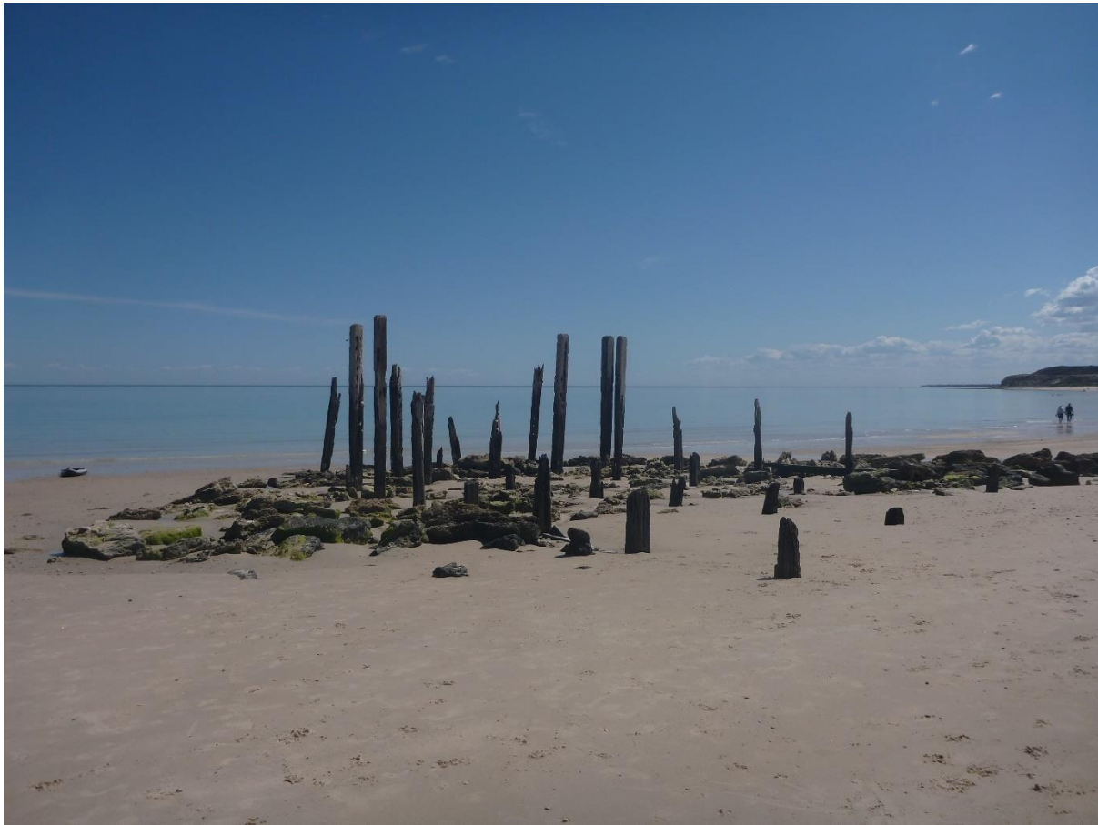
Figure 3-15 The remains of the second jetty. Photograph by P. Straiton 2019.
