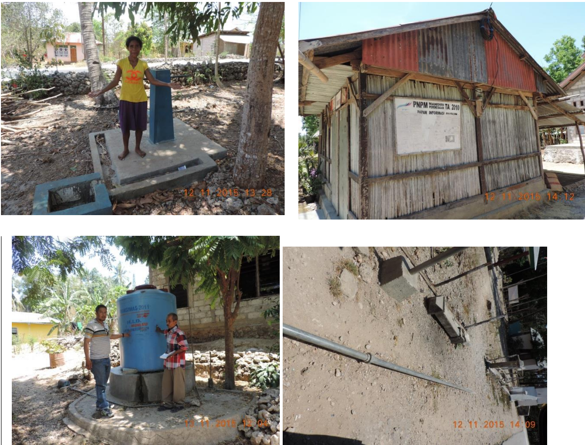
Figure 43: Neglected central government water project infrastructure (photos by author)
