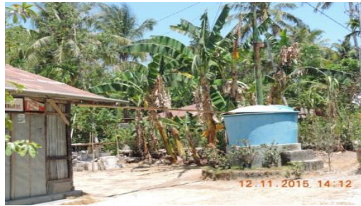
Figure 8: Rainwater harvested from roof gutters (source: researcher)
