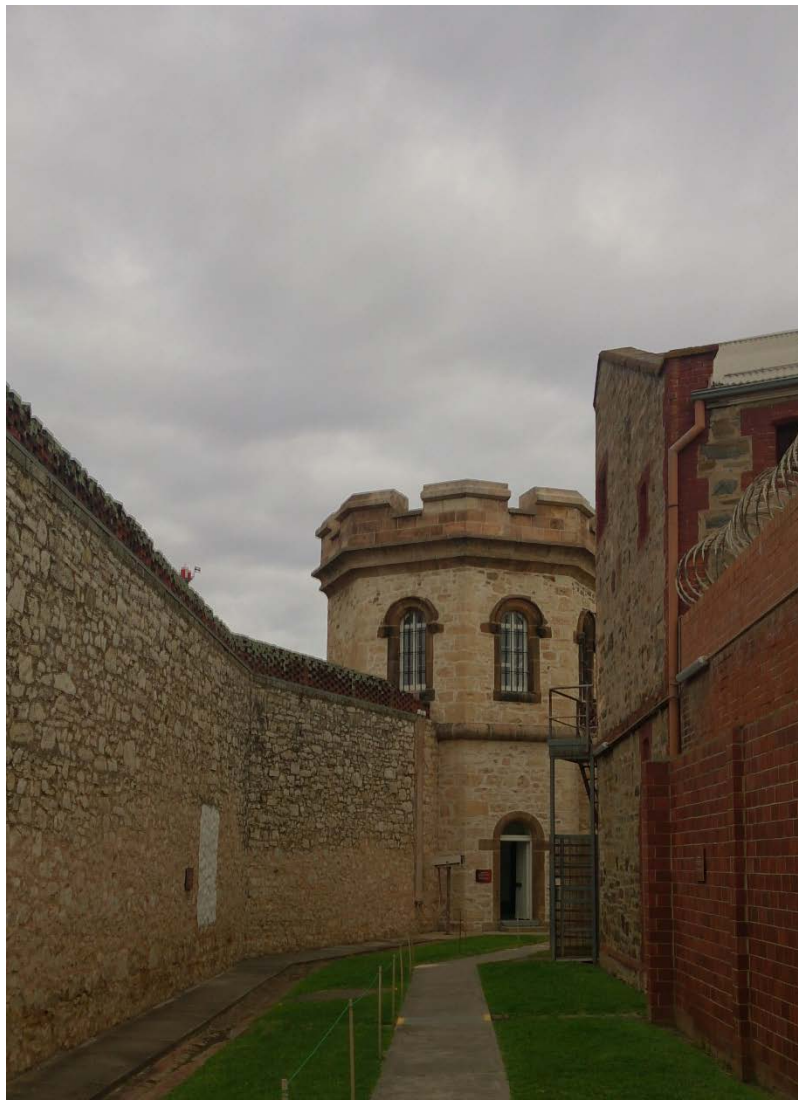
FIGURE 8 THE EXECUTION TOWER: ADELAIDE GAOL, AUTHOR
